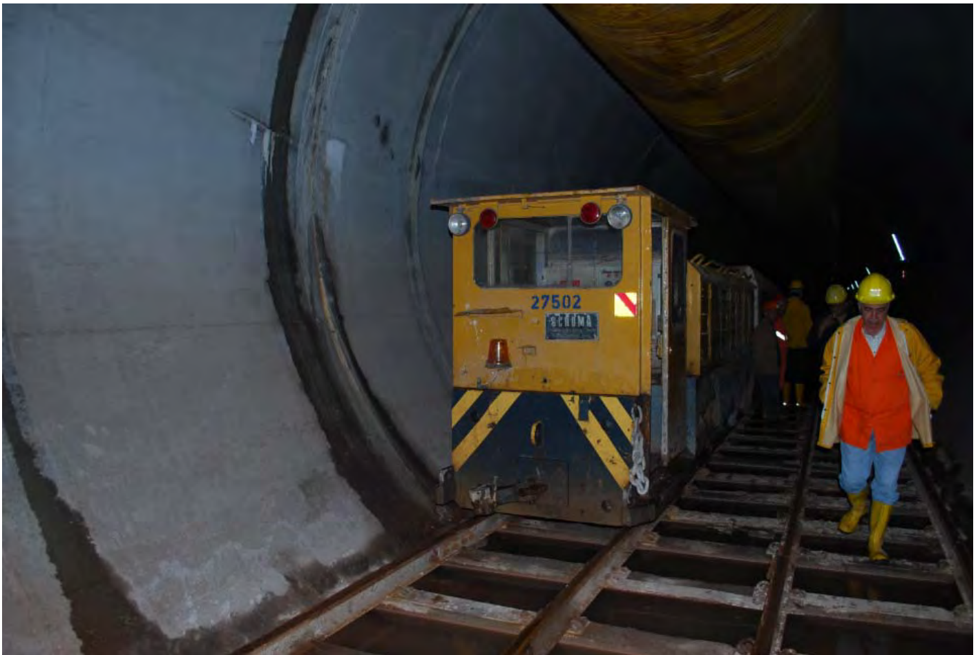
Acheloos Water Transfer Tunnel to Thessaly (17 Km length)
