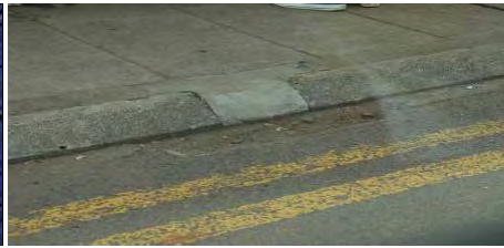
Drain with covered side inlets
