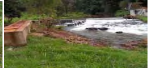
Existing irrigation dam
