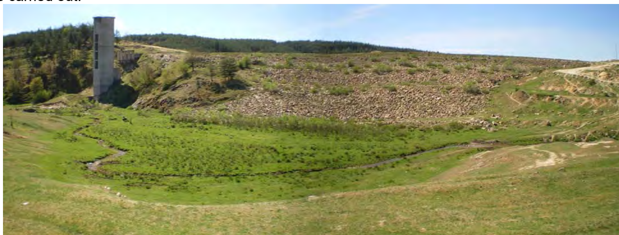
Upstream view of existing part of Luda Yana Dam
