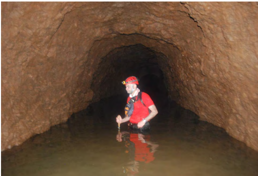
Inspection of Mathioya Tunnel (5.2 Km long)
