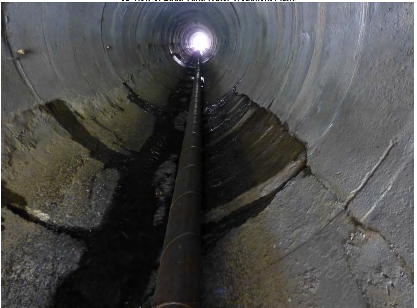
Diversion and draw-off tunnel to be fully rehabilitated
