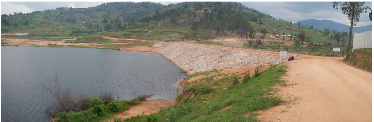
Nyanza Dam during first filling (2014)
