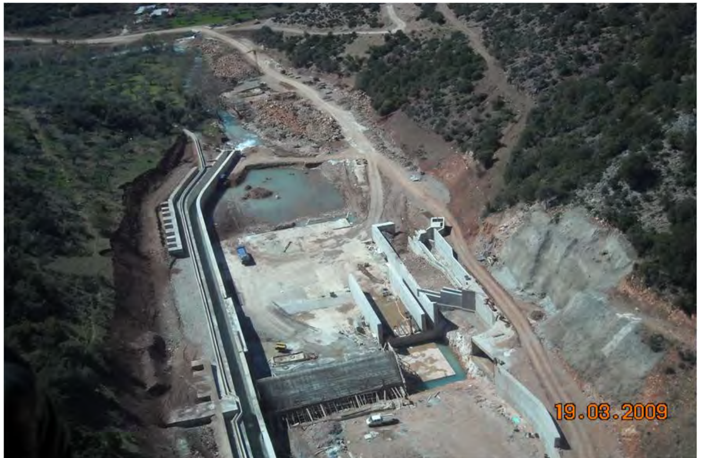
Upstream view of diversion dam
