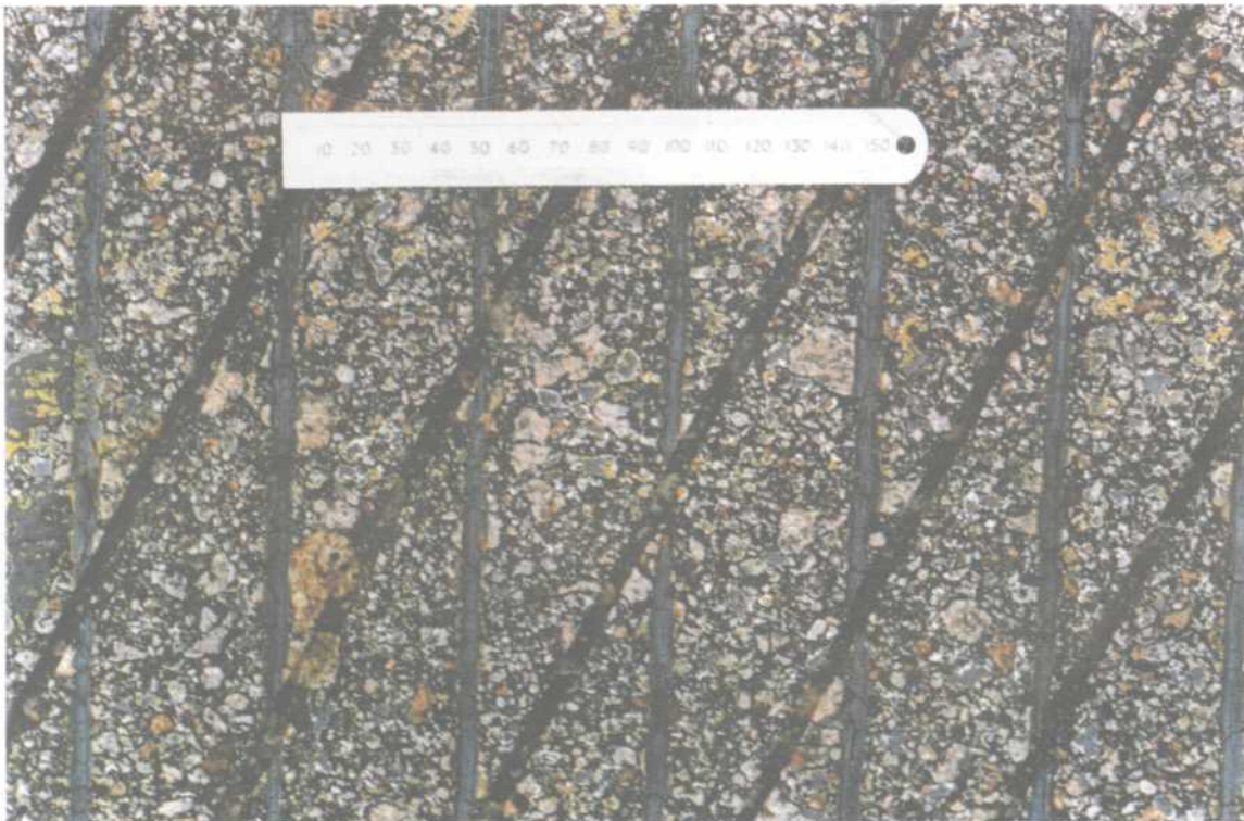
Fig 8 Cross grooving near the 31 threshold
