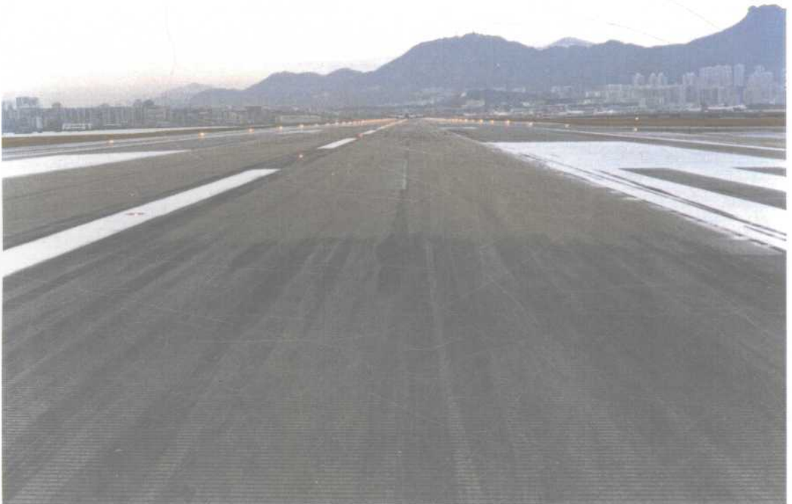
Fig 9 Effects of rubber removal
