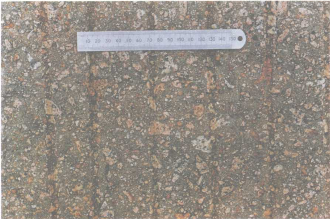
Fig 7 Close-up of worn grooves
