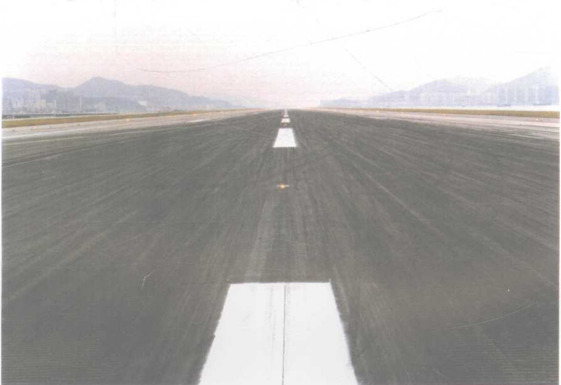
Fig 3 Close-up of uncontaminated grooved asphalt surface
