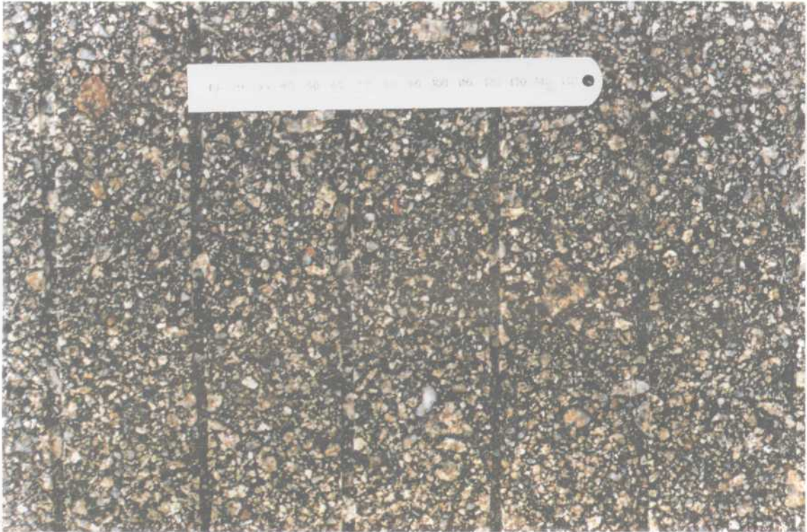
Fig 3 Close-up of uncontaminated grooved asphalt surface
