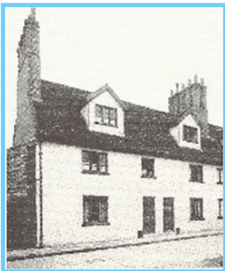
Felaw's house, prior to demolition
