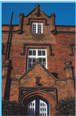
Entrance to the headmaster's residence, now the staff entrance
