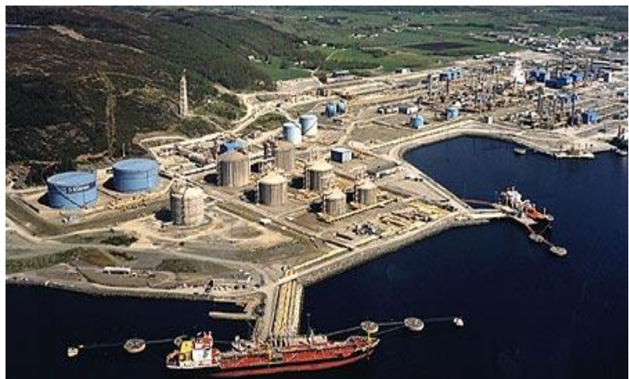
Kårstø onshore facility. Source: StatoilHydro
