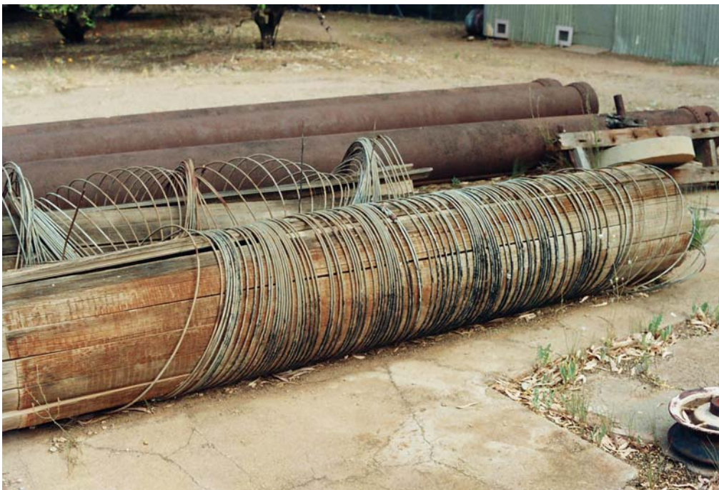
Plate 8. Sections of woodstave pipeline removed from the Umberumberka to Broken Hill gravity pipeline installed in 1915. The wires wrapped around the timber section contain the internal pressure.
