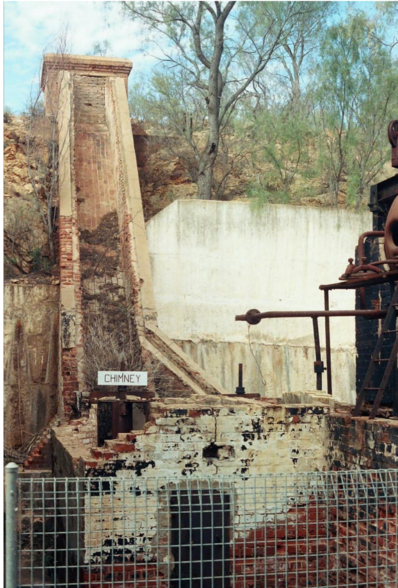
Plate 4. Umberumberka Pumping Station. Flue and Chimney Base behind boilers. The chimney was placed on the escarpment to increase its effective height.
