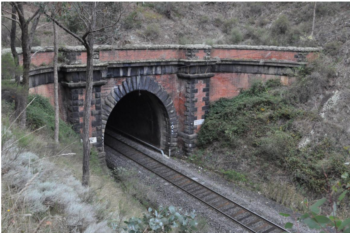
Elphinstone Tunnel (Western Portal) in 2011
