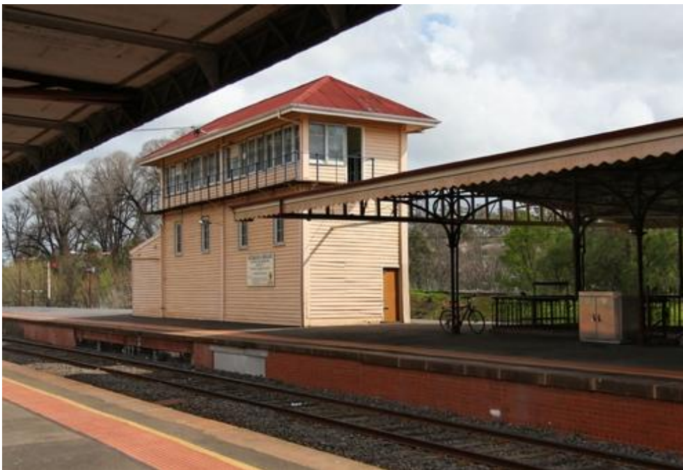
Castlemaine Signal Box and platforms.
