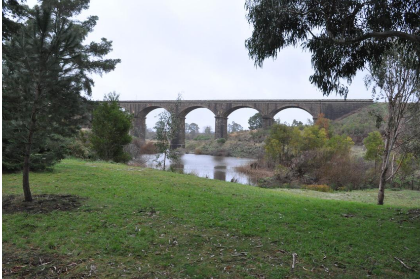
Malmsbury Viaduct in 2011 from the location where the interpretation panel is proposed to be erected in the Malmsbury Botanical Gardens
