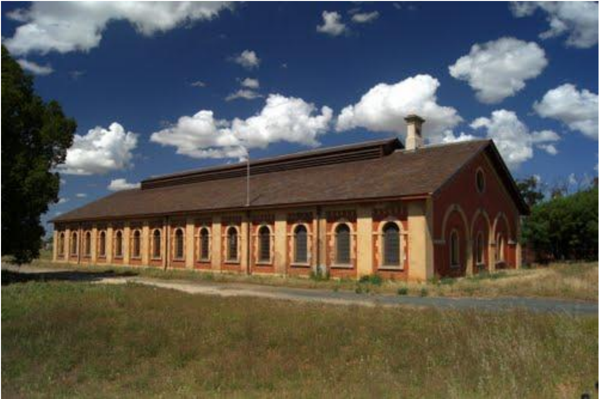
Echuca Locomotive Shed.
