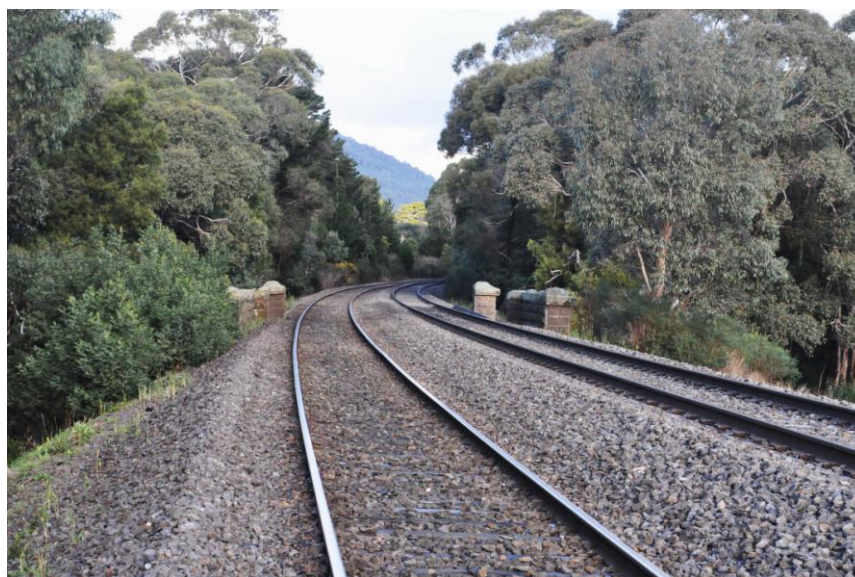
Trackwork at Woodend in 2010, looking south with a bridge over a minor road in the foreground.
