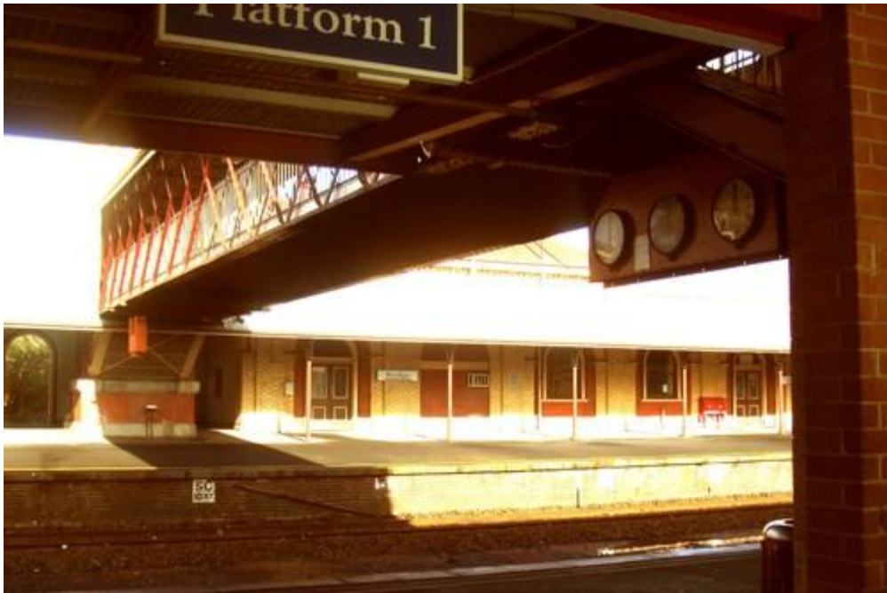
Bendigo Railway Station platforms and footbridge.
