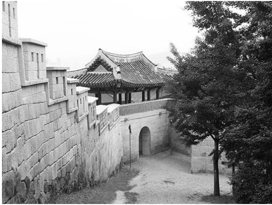
Fig. 13 North Gate of the Dongnaeupseong Fortress Site, 2009, retrieved in January 30, 2016. https://commons.wikimedia.org/wiki/File:North Gate of the Dongnae eupseong site.JPG
