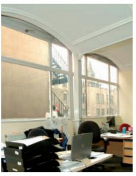
Figure 61 (above) Glazed curtain walling to the courtyard elevation of Oriel Chambers, independent of the building's cast-iron frame. [DP28852]
