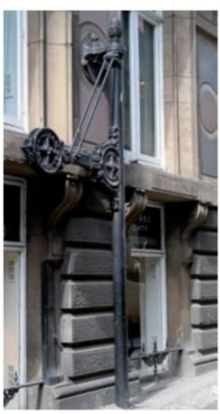
Figure 43 (above) An unusually decorative cast-iron hoist in Hackins Hey, originally serving the basement of 11 Dale Street. [Joseph Sharples]
