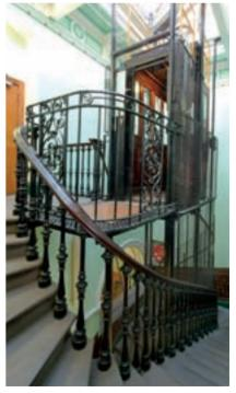
Figure 67 (right) Cast-iron spiral staircase at 16 Cook Street, c1868. [DP28731]
