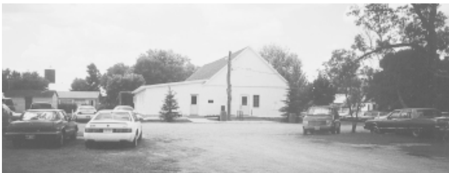
The Reinland Community Centre as seen today in Reinland, Manitoba, view to the west. This building was the Reinland Mennonite Church from 1876 to 1922 when many emigrated to Mexico. As of 1923 the Blumenort Mennonite Church used it until 1968. The church building became the Community Centre in 1970 when a kitchen was added. The memorial plaque is located at the front right side of the building, just beside the pine tree.
