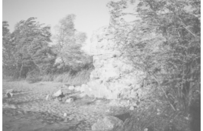
Concrete casing which once served as a well for the village of Andreasfeld.
