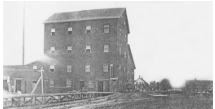
Photograph of the Barkman and Reimer flour mill in Steinbach constructed on Mill Street (now First Street), after the first mill was destroyed by fire August 16, 1892. Note the buildings of flour mill shareholder and manager Johann I. Friesen in the background (“Schloss Kinder Reich”), situated where the new “Stone Creek” condominium was constructed in 1999. View towards the southwest. These buildings were later purchased by Peter B. Reimer who married “Malla Fries’ Katharina”. Compare with the photo in Preservings, No. 9, Part Two, page 44.
