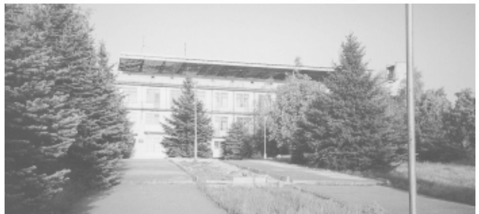
"Progress" the Rehabilitation facility at Andrejewka, view from the beach.
