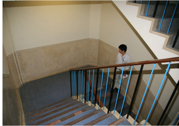
Typical staircase in the East Wing
