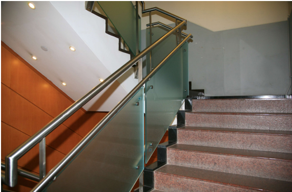
The contrasting finishes to the east stair in the West Wing
