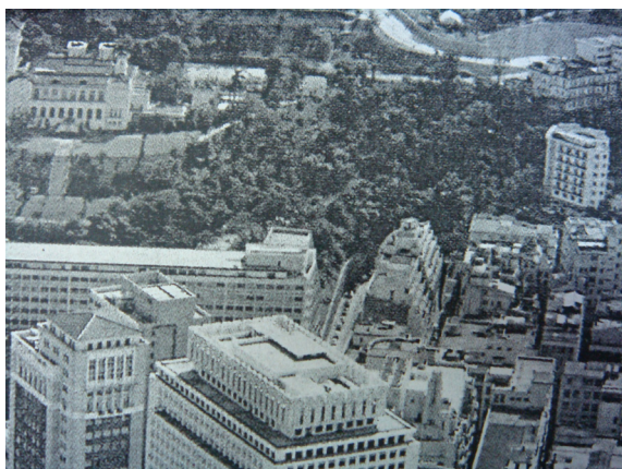
View of the West Wing in the 1970s showing the stepped back facade of the building opposite (Moss, 2002, p.165)
