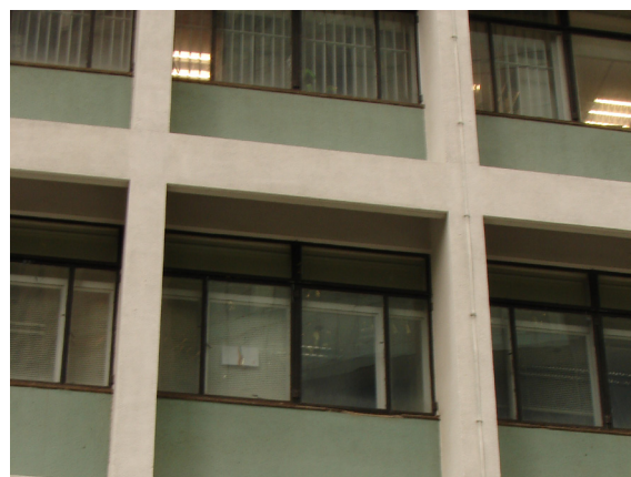
The exposed concrete frame and steel windows of the CGO
