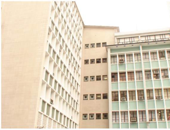
The granite clad 'transitional' section of the East Wing, elevation 1
