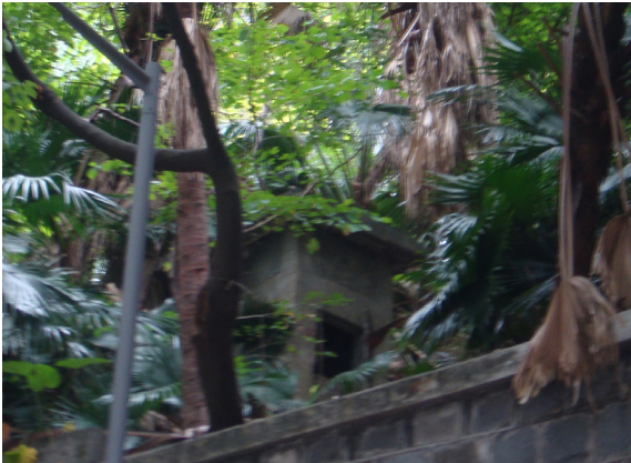
The ventilation shaft on Ice House Street
