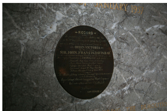
The circular metal plaque from the foundation stone of the Old Government Offices
