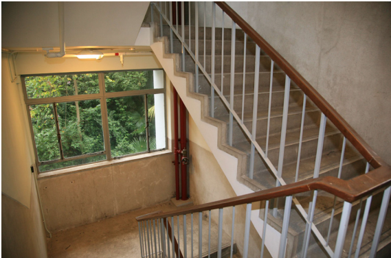
The southwest corner staircase in the West Wing
