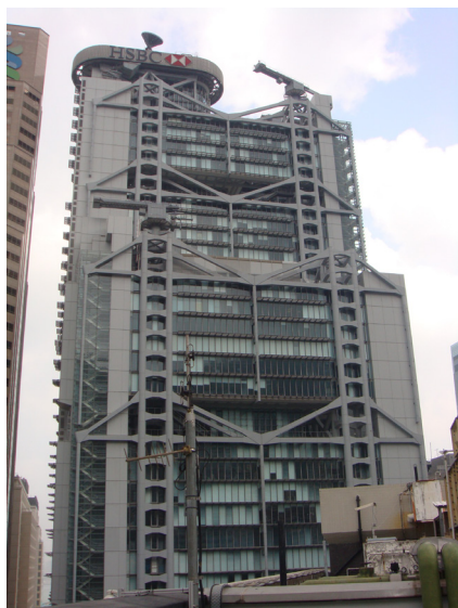
Norman Foster's HSBC building as seen from the CGO compound
