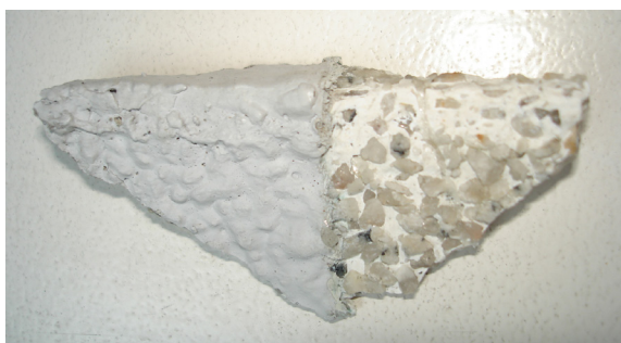
A sample of the concrete from the West Wing
