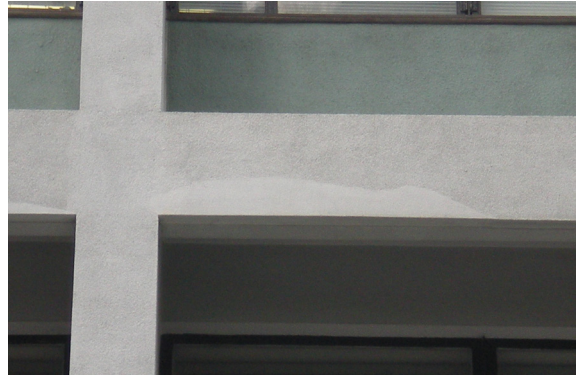
Concrete repairs to arrisses
