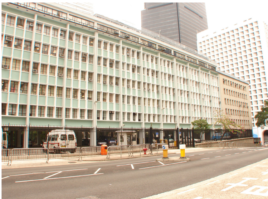
The main central section and the eastern section of the East Wing, elevation 1
