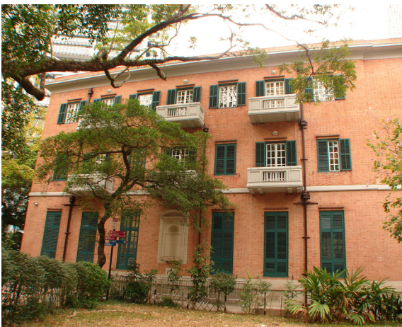
The south elevation of the French Mission Building
