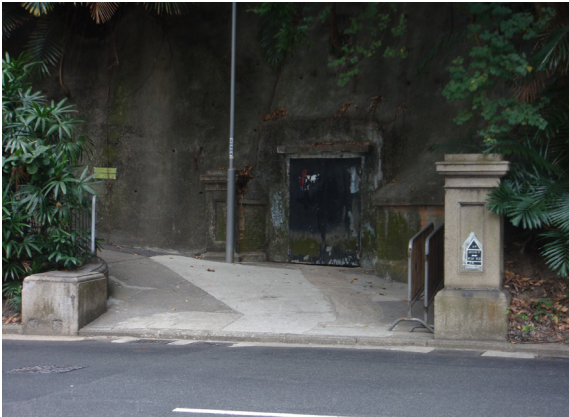
The western portal on Lower Albert Road
