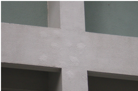
Concrete repairs on the West Wing
