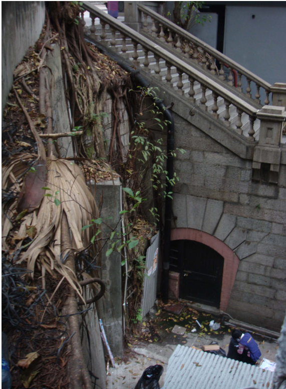
The tunnel portal under the Duddell Street steps
