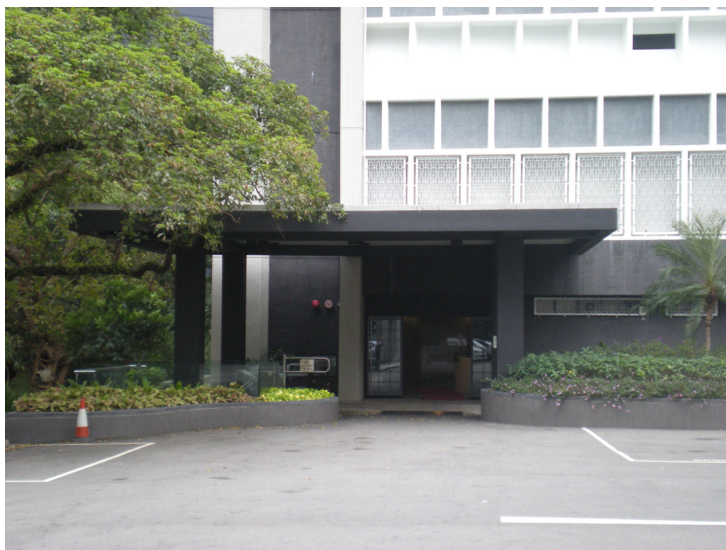
The canopy over the New Annexe entrance
