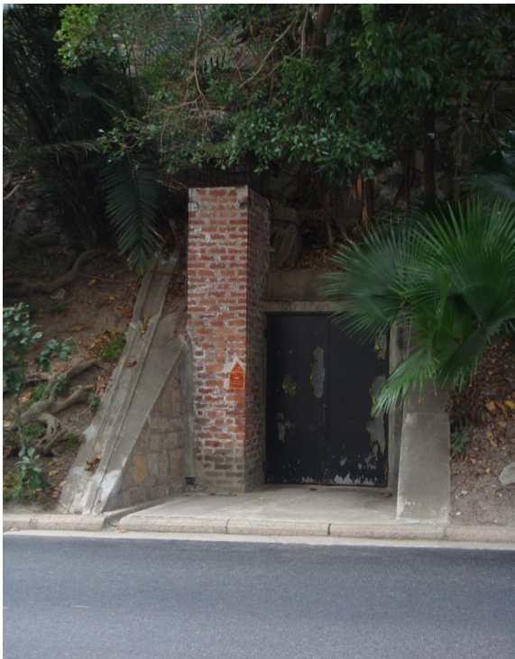
The eastern portal on Lower Albert Road
