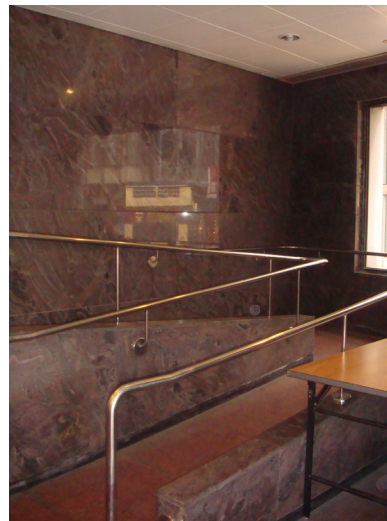
The access ramp in the ground floor reception of the West Wing
