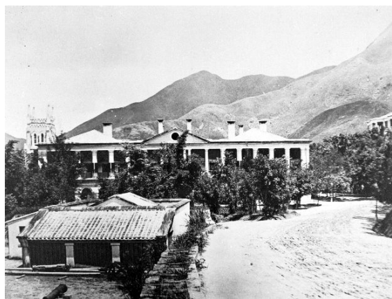
Early photograph of the Old Murray Battery with the Government Offices in the background
