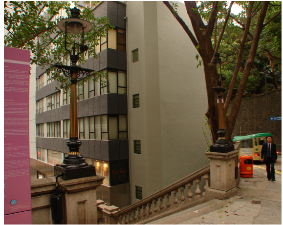
The Duddell Street steps and gas lamps
