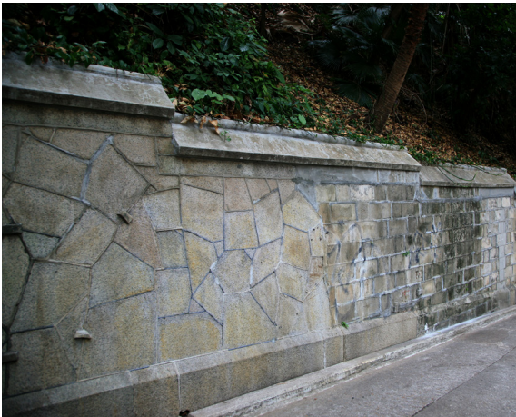
The retaining wall on Battery Path
