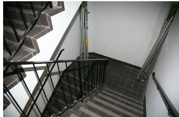
The escape stair in the Central Wing
