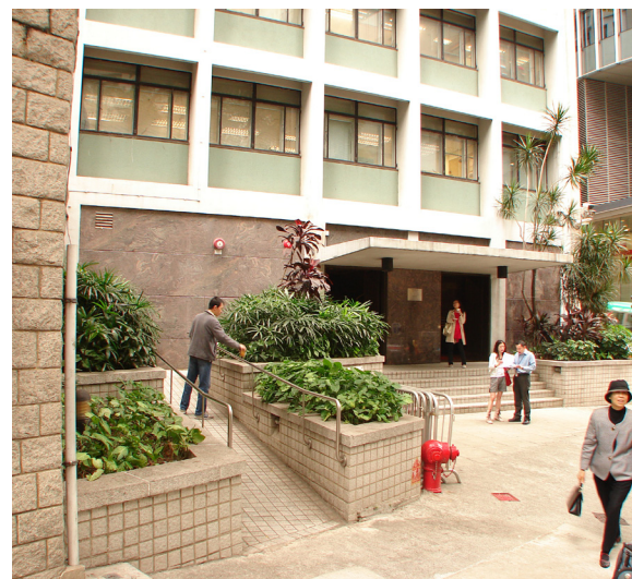
The west entrance to the West Wing
