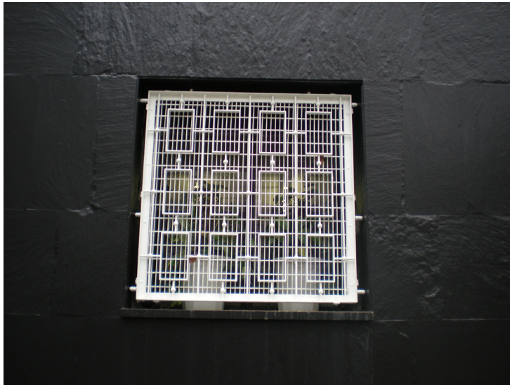
Painted slate on the ground floor
