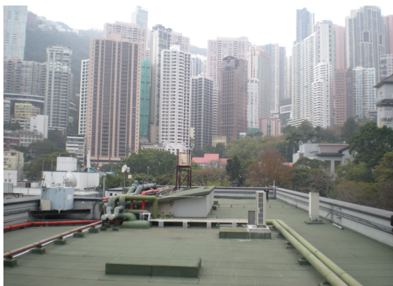
The roof of the Central Wing
