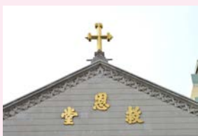
教堂正面的山牆附有裝飾簷板 Pitched gable façade with decorative verge boards and ornaments
