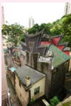
「五岳朝天」式山牆 Gable walls in "Five Peaks Paying Tribute to Heaven" style
