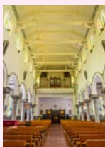
教堂以鋼筋混凝土建成，外形上模擬中式木建築梁架結構 The church was built in reinforced concrete and its truss resembles the structural features of Chinese classical architecture
