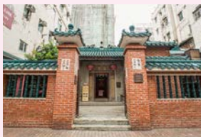
廟前空地有兩道以綠色琉璃瓦蓋頂的紅磚矮牆連柱 Open space in front of the temple surrounded by two red-brick low boundary walls with columns, both are topped with green glazed roof tiles
