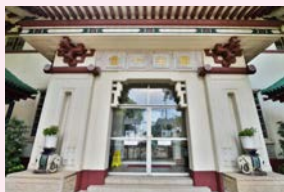
斗拱上置飾有中式圖案的挑簷桁 Above the bracket sets or dougong are cantilever purlins decorated with Chinese motifs
