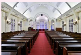
二樓的羅馬式圓形橫拱支撐金字屋頂，並由三個半圓形拱門分隔聖壇和正殿 Romanesque rounded transverse arches on the second floor supporting the pitched roof. Three semi-circular arches separating the nave from the chancel
