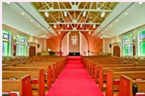
以瓦片、木梁及鋼架建構的金字屋頂 The pitched roof built with clay tiles, wooden rafters and steel trusses
