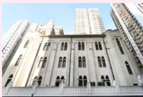
教堂所有立面每層均有尖頂窗，部分對稱成組 All of the elevations fenestrated with lancet windows at each level, some of which are paired
