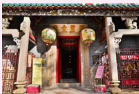
前殿前檐由一組精緻雕刻的花崗岩石柱和木梁架支撐 Front eaves of the front hall supported by a system of granite columns and lintels
