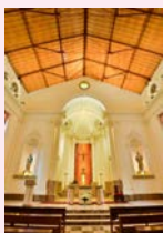
後殿上置半圓穹頂， 而正殿則為金字頂 A dome over the apse and a pitched roof over the central nave
