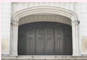
在都鐸風格的扁平拱內有三道以三葉飾和四葉飾點綴的木門 Tudor style entrance with a flattened arch embracing three timber doors decorated with trefoils and quatrefoils
