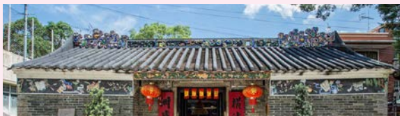
前殿正脊飾有「鯉躍龍門」為題的灰塑 Main ridge of the front hall with an auspicious theme of "Carps jumping over the dragon gate" plaster mouldings
