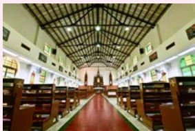
屋頂內部可見鋼架結構 The steel roof trusses are exposed
