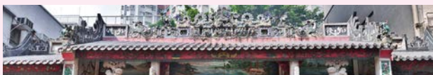
前殿正脊飾有灰塑和石灣陶塑，檐板則飾有花卉和吉祥圖案 Main ridge of the front hall with plastered mouldings and Shiwan ceramic figurines, while eave boards decorated with floral and auspicious motifs
