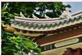
屋面以綠色琉璃瓦和素瓦鋪砌而成， 戩脊上則飾有白鴿 Roof covered with green glazed and plain tiles, while corner ridges decorated with pigeons figurines
