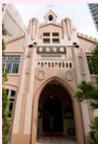
門廊的牆面飾有哥德式尖拱及四葉飾 The wall of the porch decorated with Gothic arches and quatrefoils
