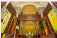
由幾何圖案彩色玻璃所組成的圓拱形窗戶及木門 Round-arched windows and doors glazed with small panes of stained glass in simple geometric patterns
