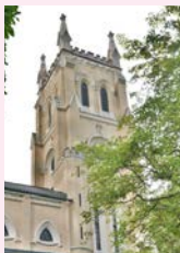
塔樓上的垛口式女兒牆和角塔 Crenelated parapet on the tower and flanking turrets
