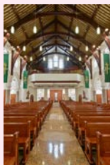
屋頂由半圓形木桁架結構支撐 Roof supported by a dome-shaped frame structure
