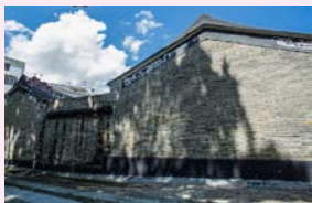
青磚建築，山牆飾有花葉為題的灰塑 Green brick structure with wall friezes in leafy and floral plaster moulding decorations
