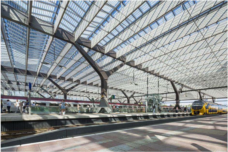
Figure 18. Rotterdam Central Station glass roof above platforms, image source: Jannes Linders
