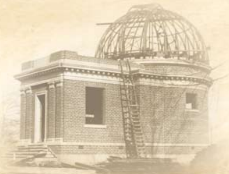
Mitchel Building under construction 1904
