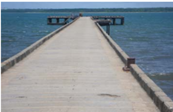
Port of Daru Pier
