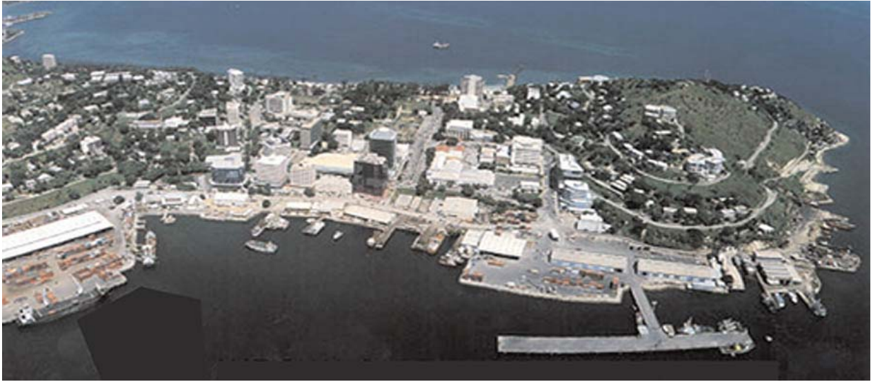
Port Moresby—Main Wharf facing SE
