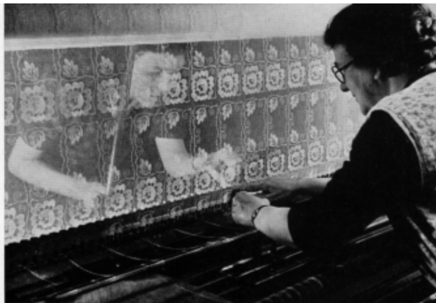
The design being traced by the pantograph operator in the picture at left is here seen being embroidered on to the net. It is the movement of the net through various planes in sympathy with the pantograph which completes the design. The operator makes one movement of her master pointer for each stitch. The operator in front is traditionally known as the Front-Girl. She mends the yarn if it breaks. The Back-Girl, just visible through the lace, attends to the shuttles.
