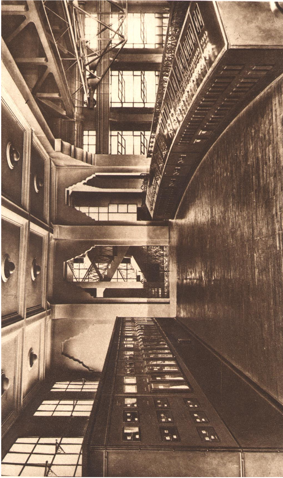
THE SWITCH ROOM IN THE GENERATING STATION
