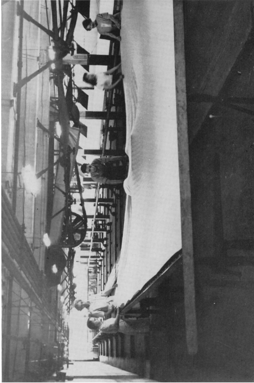
Pinning the web on the dressing frame
