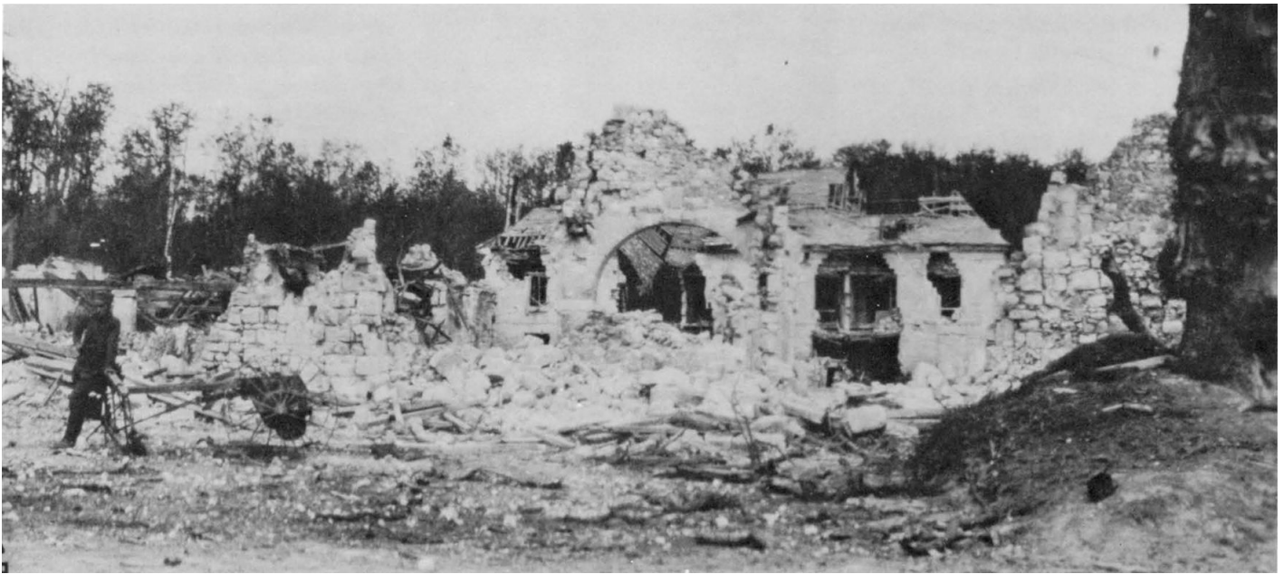
Except for an elegant arched entrance, the Verte Feuille farmhouse in the 2d Battalion's zone of action is wrecked by the heavy fighting and shelling of mid-July 1918. The 45th Company with about 100 Marines—half-strength—was sent there to the aid of the battered 55th Company, whose officers were all casualties. The 45th came away from the farm a third less again in number.
