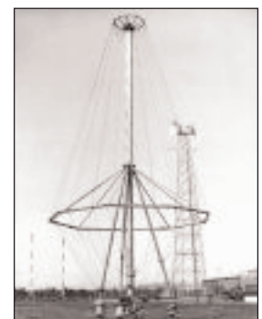
Cox Peninsula Transmitter
