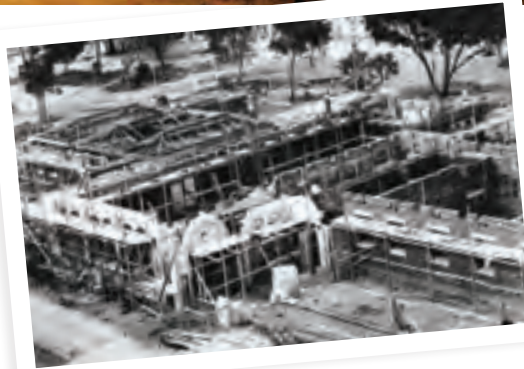
The Hackett Memorial Buildings under construction (Photo: UWA Archives)
