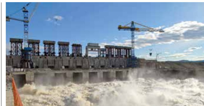
Construction of Ust-Srednekan HPP
