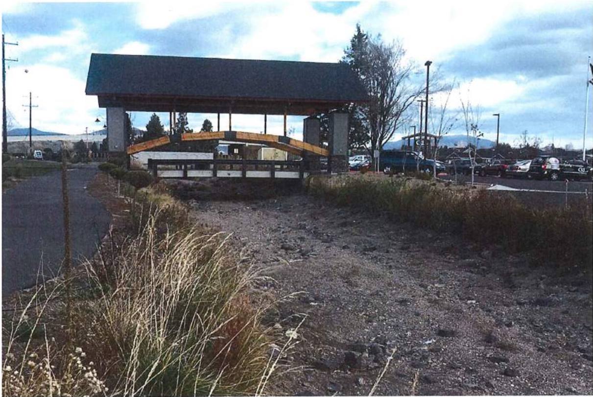
Photo 33 of 49: Pilot Butte Canal: Downtown Redmond Segment Historic District, Medical Center bridge, looking northeast
