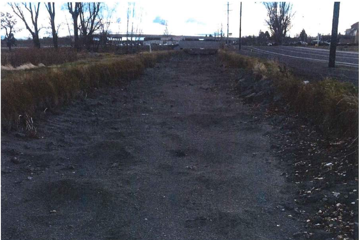
Photo 44 of 49: Pilot Butte Canal: Downtown Redmond Segment Historic District, looking south from 2036 NW Canal Boulevard bridge
