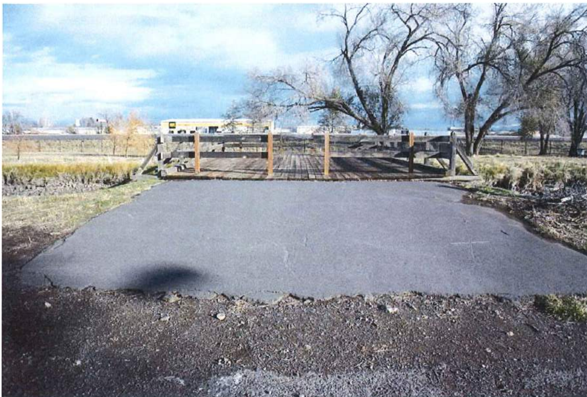
Photo 15 of 49: Pilot Butte Canal: Downtown Redmond Segment Historic District, NW Greenwood Avenue bridge, looking east
