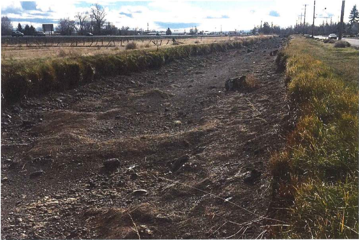
Photo 27 of 49: Pilot Butte Canal: Downtown Redmond Segment Historic District, looking southeast to NW Hemlock Avenue bridge
