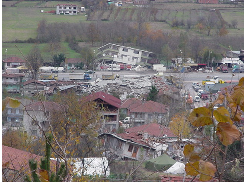
Figure 18(a) View of Merkez District, Kaynasli, looking north (N40.4629, E31.1931)
