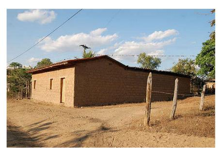
Figure 6. Adobe houses rebuilt following the local tradition in Ocotal, Nicaragua.
