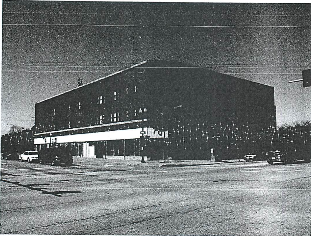
Figure 23. 701 W. Main St., Peoria, Illinois. NW corner of Main St. and SW Perry Ave.
