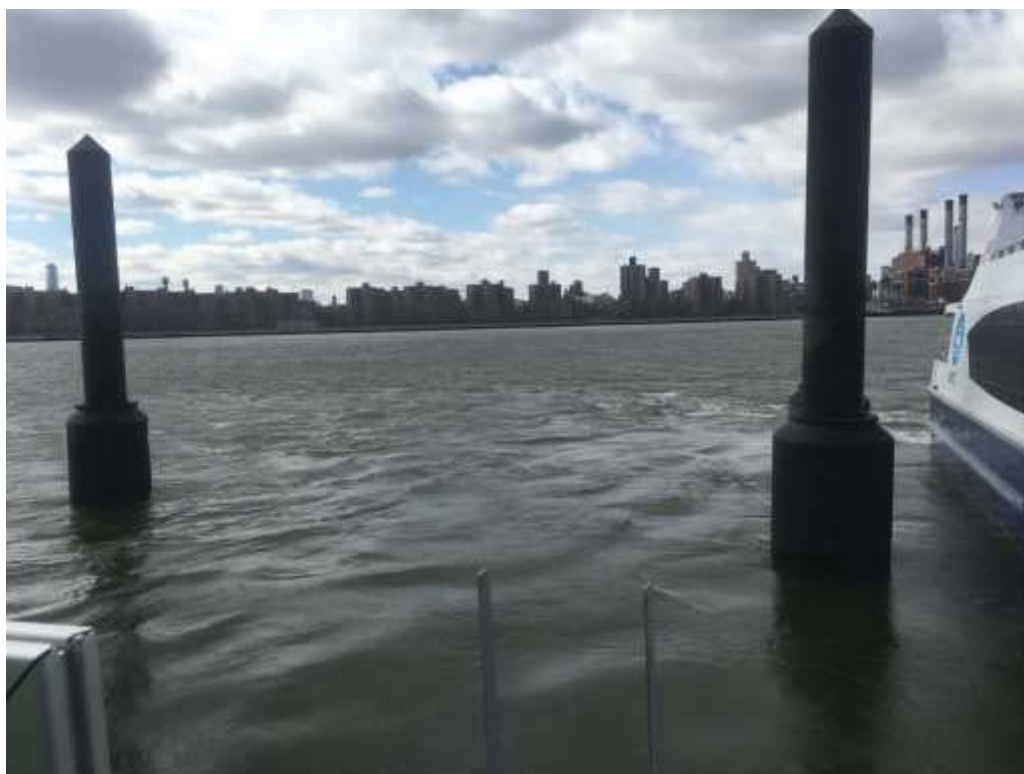
Photo B: View of East River facing east toward Manhattan at location of existing ferry pier to the south of proposed project location.
