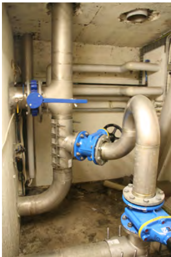
Figure 3. The new pipe bypassing the biogas dome, photo by Thorbjörn Rydén.
