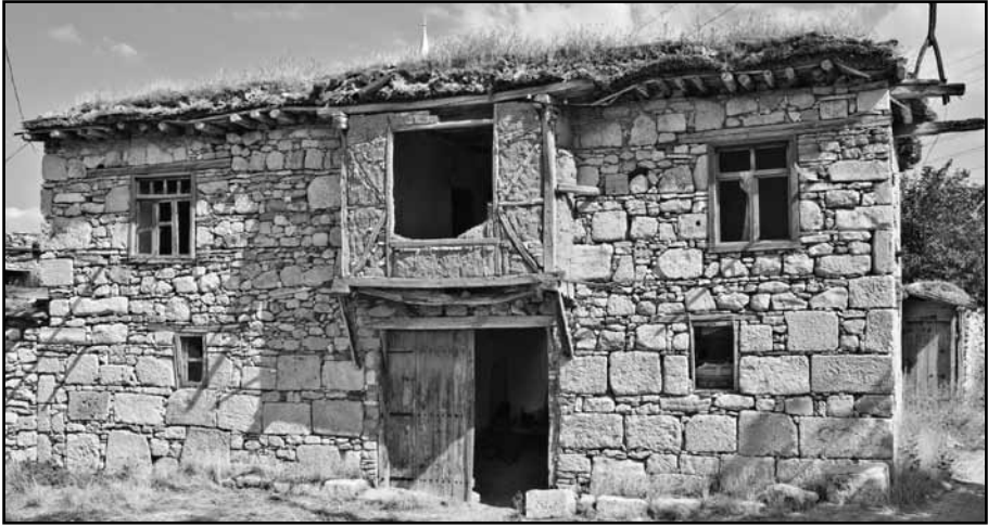
Fig.14: Turkish house, facade from west
