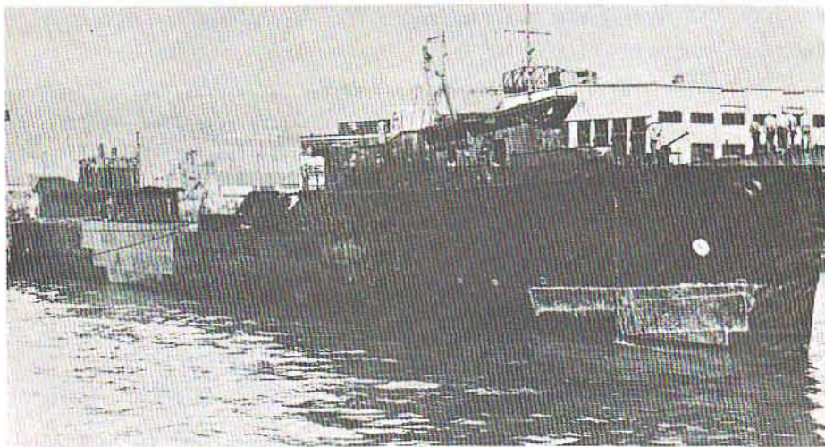
USS Downes afloat, being removed from drydock, 6 February 1942. Note wrinkled plating.
