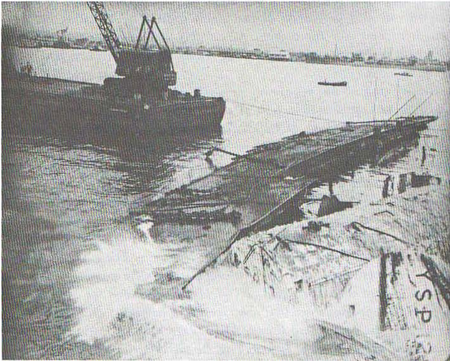
Pontoons surfacing near bow of Oglala, 11 April 1942.
