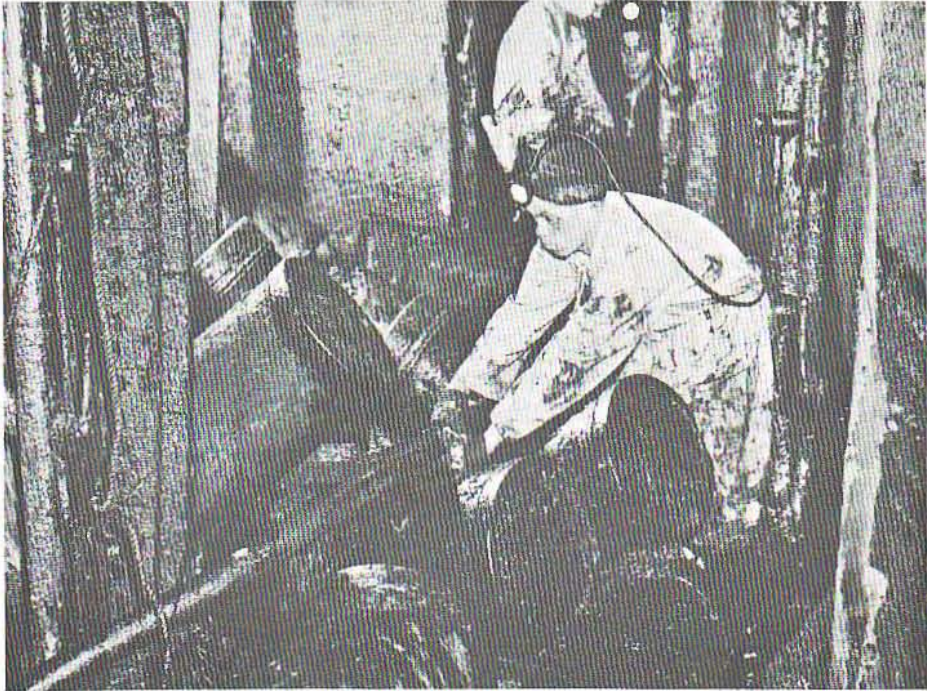
Adjusting discharge hose from submersible pump in 14-inch magazine spaces during refloating operations in Oklahoma.
