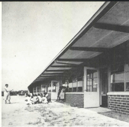
In the exterior and interior views of the typical classroom (left and below) the economical exposed structure is apparent—the steel frames 8' oc, with cantilevered outriggers along the south windows; exposed structural-acoustical roof decking; plywood partition between rooms.
