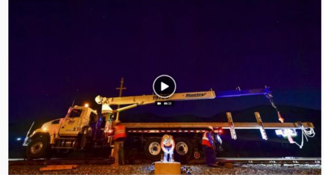
POLE INSTALLATION: TIME-LAPSE VIDEO
