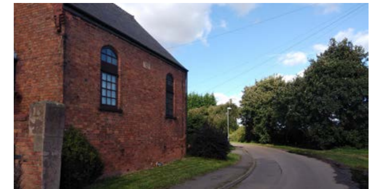
Fig 66: Constructed in 1857, the old Methodist Church is a modest but charming structure..
