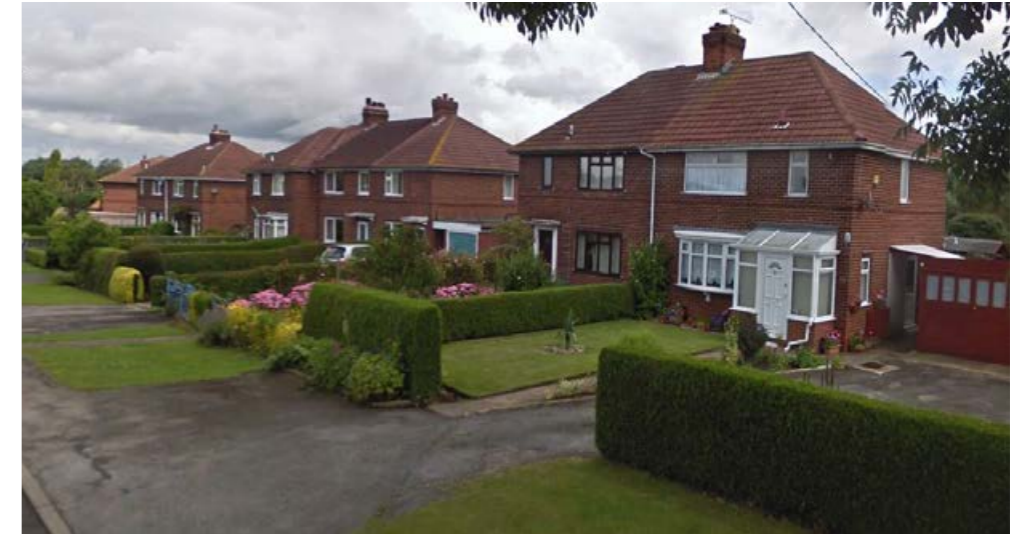
Fig 30: Though pitched roofs are common throughout Treswell, there are several occasions where hipped roofs have been preferred, such as at Cocking Lane, where the adoption of red brick and pantile roofing has helped these buildings fit in despite their more unique form.
