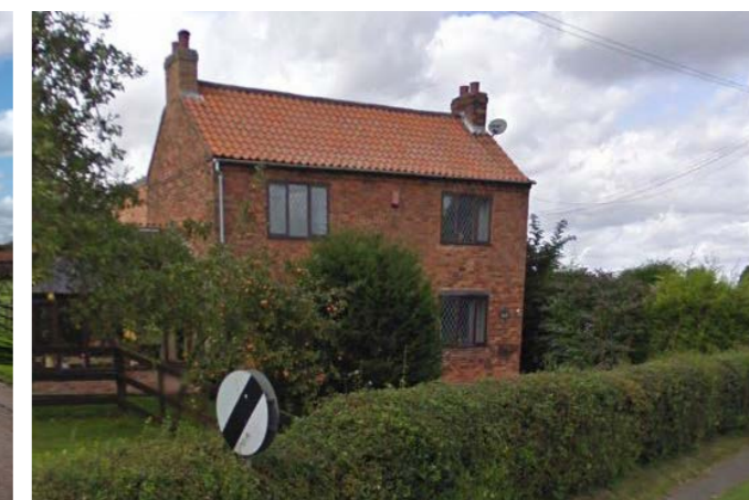
Fig 47: Two-storey detached dwellings with pitched pantile roofs accommodating chimneys and red brick walling are the most locally distinct building typology seen in Cottam.
