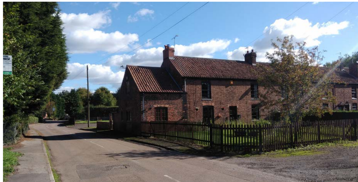
Fig 49: The extensive and handsome red brick facade of May Cottage and Ivy Cottage is one of the most striking buildings at Cottam's southern end. Topped by a pitched clay pantile roof, which is punctuated along the ridge by brick chimney stacks, and with a well-portioned facade with regular window and door arrangements, these cottages represent one of Cottam's finest pieces of local vernacular architecture
