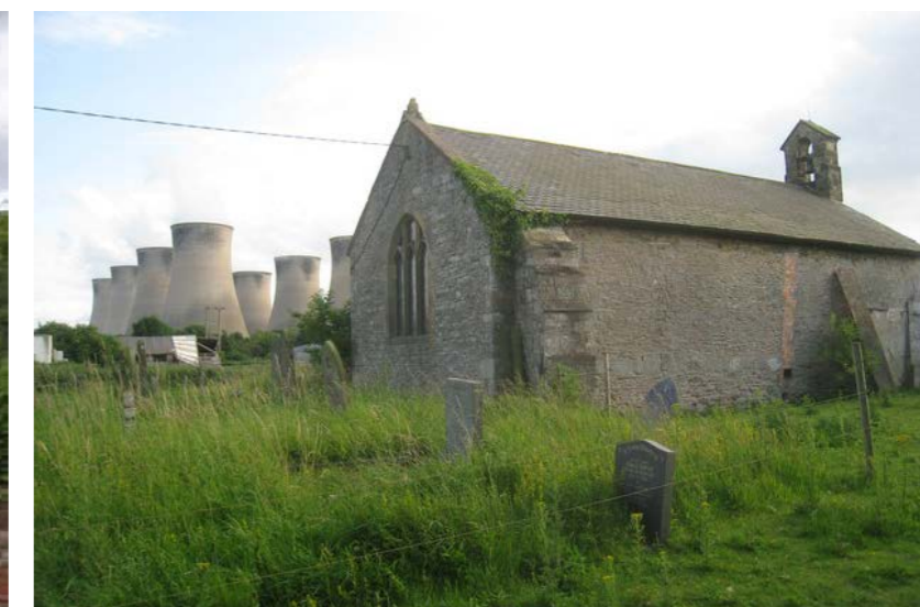
Fig 54: The Church of Holy Trinity is located to the west of the village's central spine within an open and exposed rural landscape. It is constructed of coursed rubble and dressed stone with ashlar quoins and dressings.
