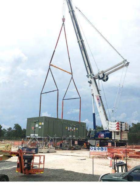
The substation switch-room arriving on site
