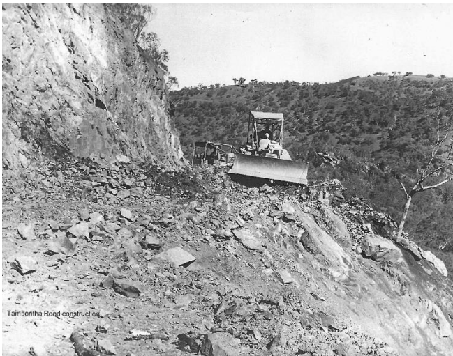
Tamboritha Road construction— circa 1960. Source Geoff Kennedy.
