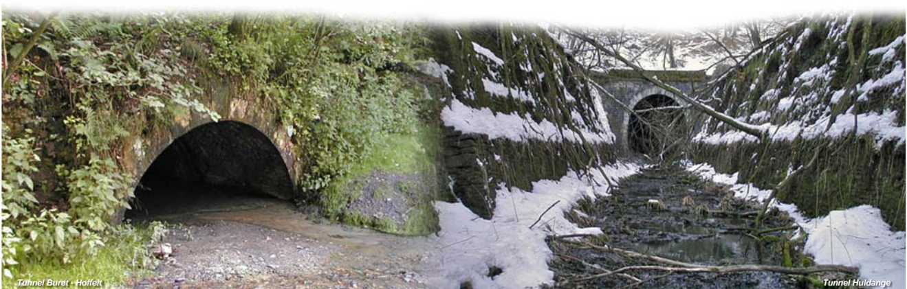
Tunnel Buret - Hoffelt
