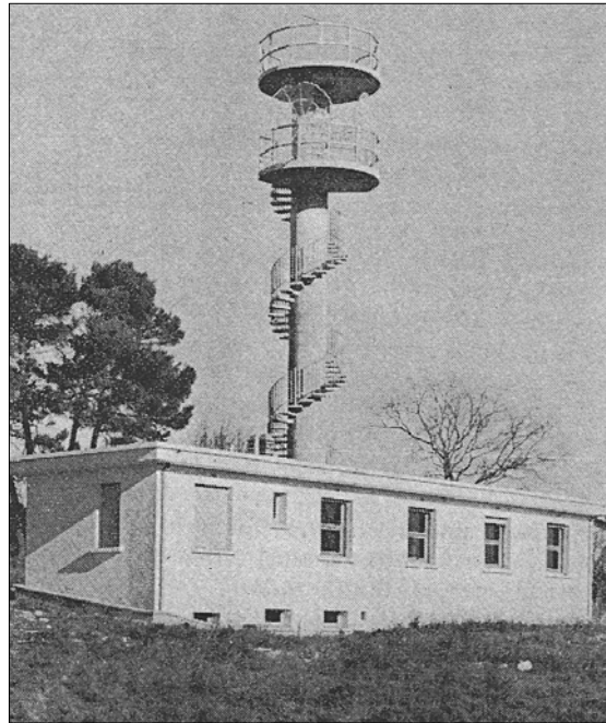
Figure 42: The central receiver building, and microwave link tower (after Laffineur and Coupiac, 1967: 394).
