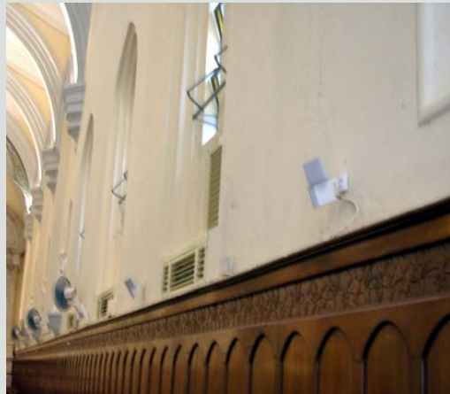
Speakers arrangement with consideration of audio requirement and its effect on interior space
