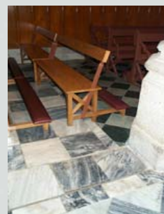
Strip of existing tiles were preserved as
