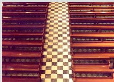
Different paving between walkway (black and white marble tile) and seating area (green ceramic tile)
