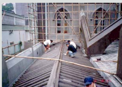
Application of SUNTEX waterproofing system
