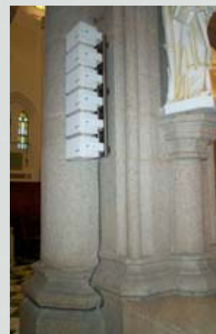
Concept of the stainless steel speaker support is to imitate the pipe organ of the Cathedral. With the protruded pipes being cut short after mock-up inspection to make it less obtrusive
