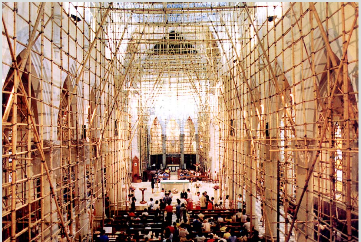
Interior view of scaffolding erection during conservation works.
