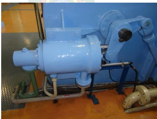
Fig.9 – Servo Motor Deflector.
