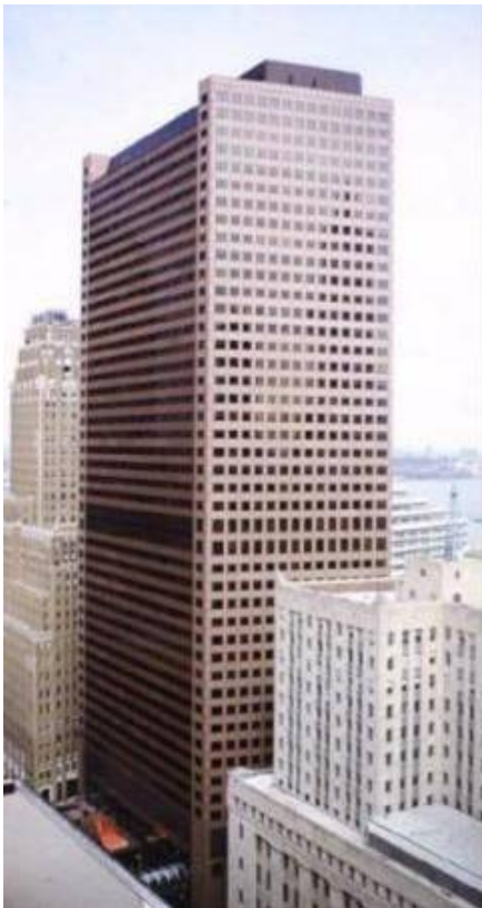
WTC 7: 47 - Story, steel-frame building..
