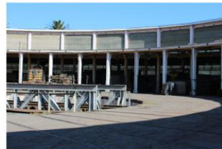
(23) Interior Tornamesa MSE (MH y ZT).
