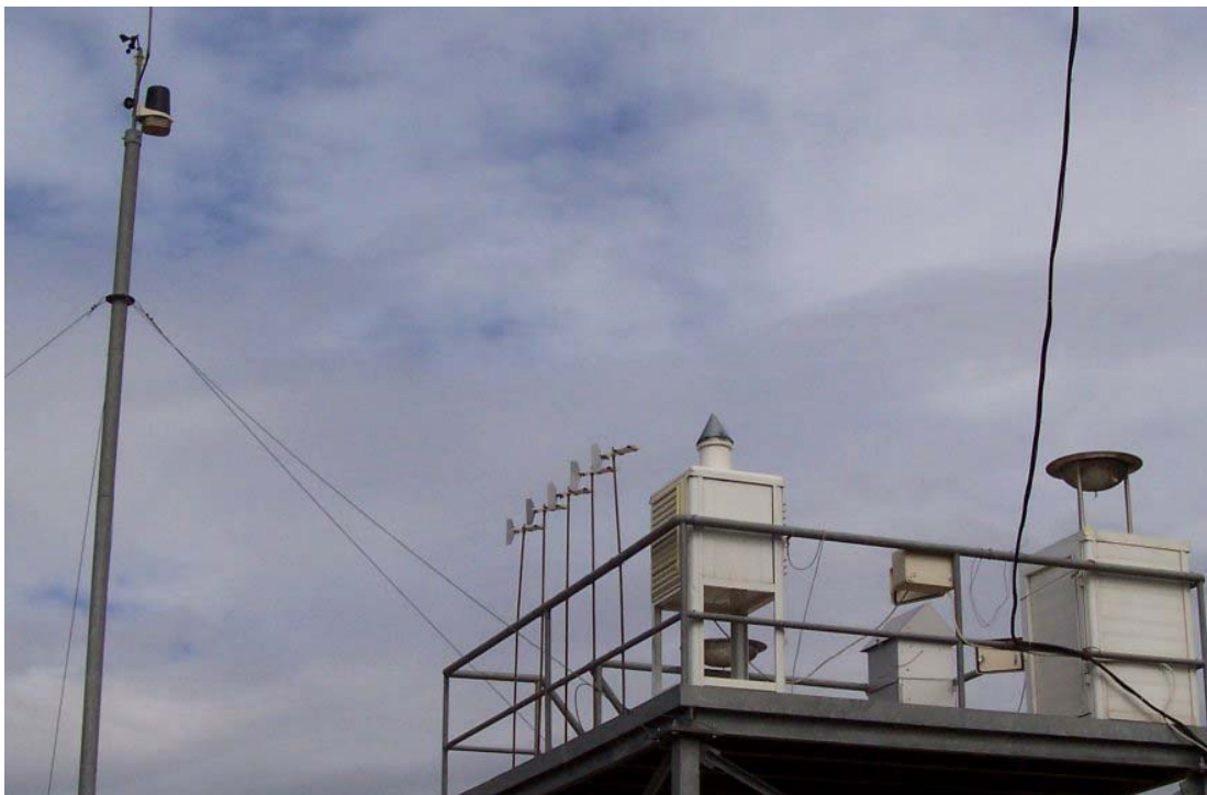
Figure 3.2 View of the sampling platform, sampling equipment and the meteorological tower
