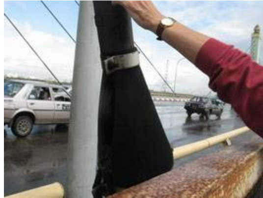
Photo-4.51 Wound cable rubber guard
