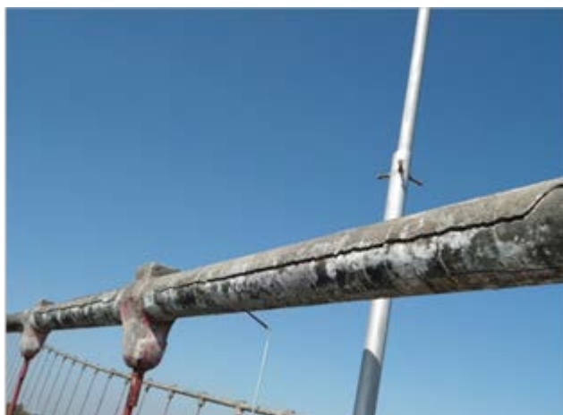
Photo—4.38 Main cable cladding
