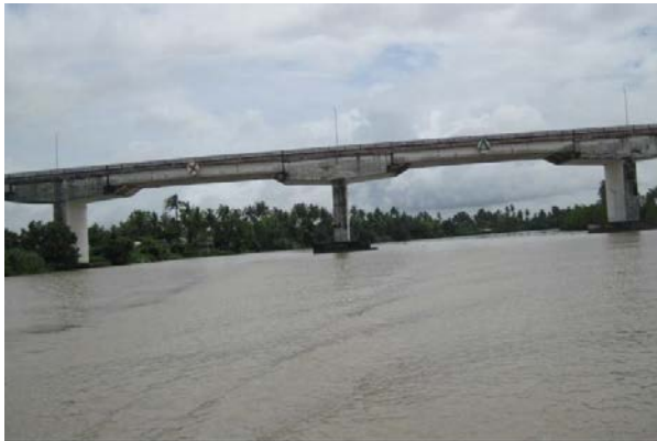
Photo-4.48 Same type bridge as Dagon Bridge
