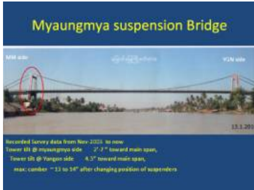
Photo-4.17 Myaungmya Bridge
