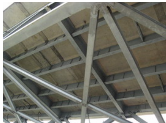
Photo-4.44 Precast concrete slab
