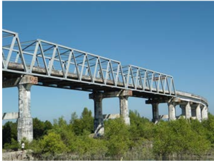
Photo—4.75 Min Kyaung Chaung Bridge
