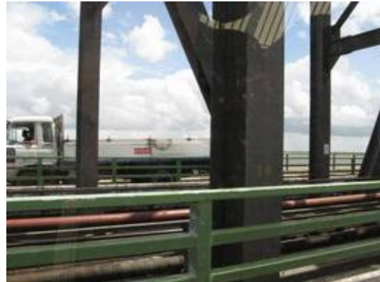
Photo-4.7 Thanlyin Bridge
