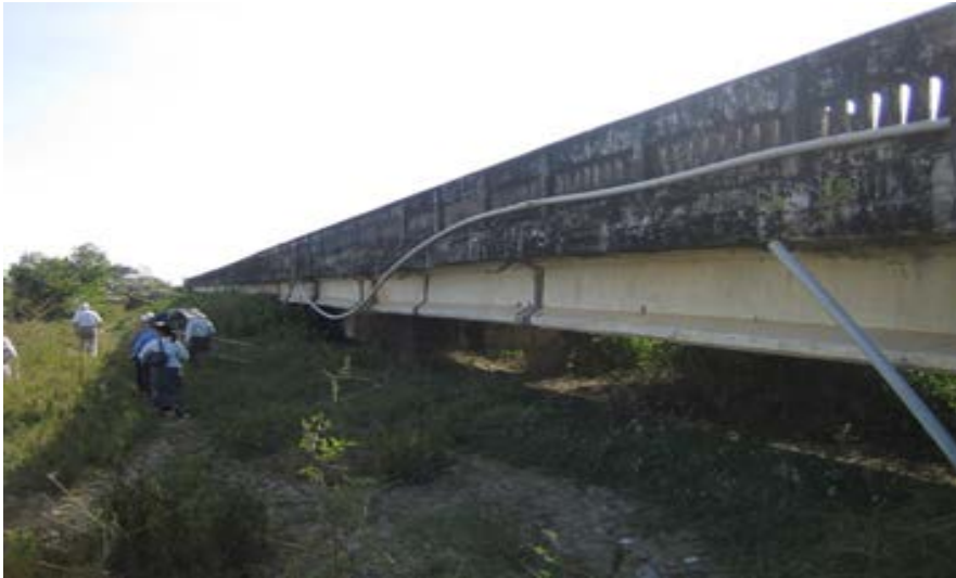
Photo—4.3 Thakhut Bridge
