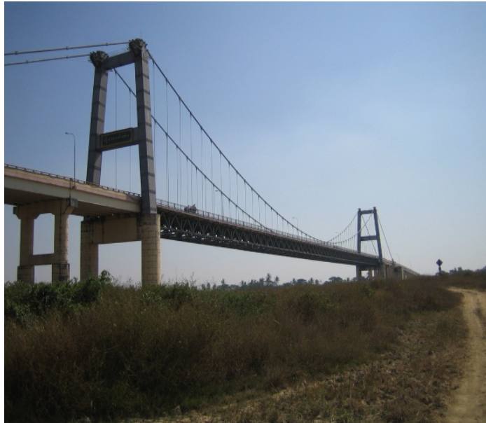
Photo—4.78 Twantay Bridge
