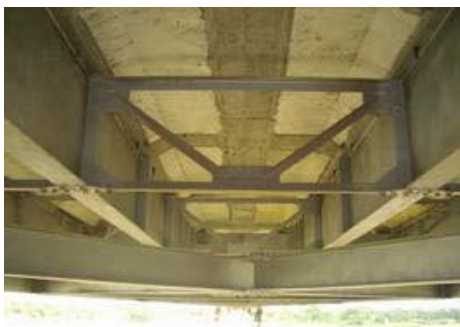
Photo—4.30 Precast concrete slab
