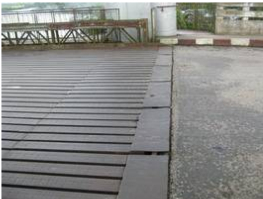
Photo-4.23 Expansion joint
