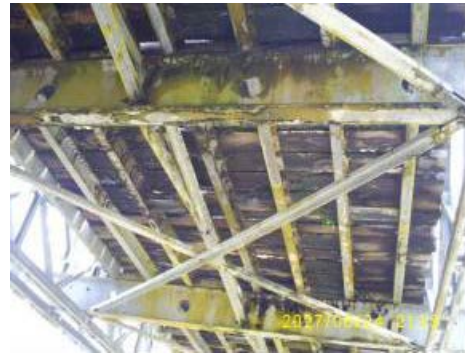
Photo-3.8 Structure of the deck
