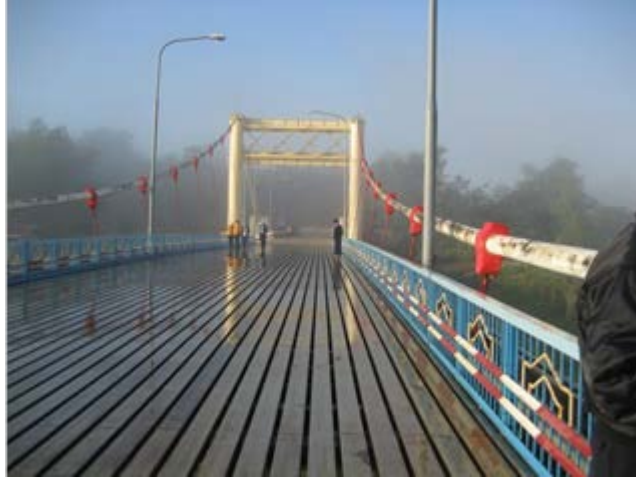
Photo—4.86 Tha Yu-Pa - PA done Bridge
