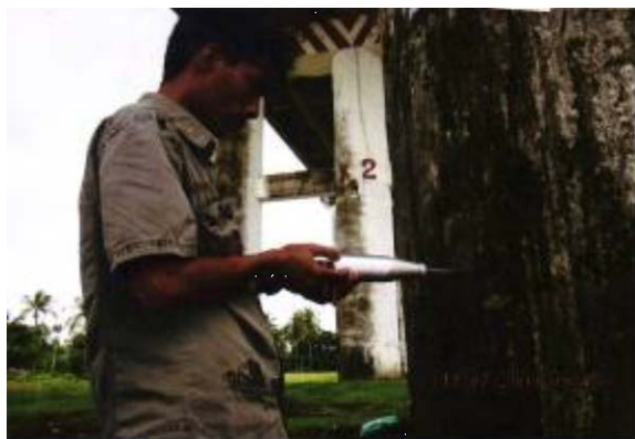
Photo-3.14 Survey using a Schmidt Hammer
