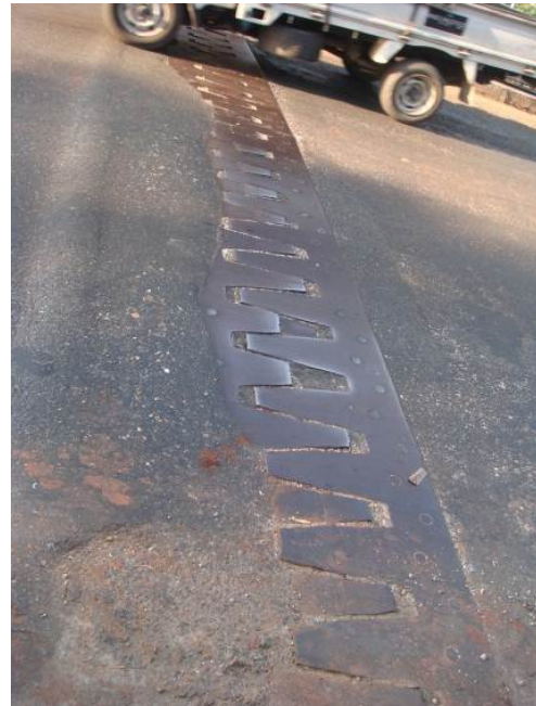
Photo-4.12 Expansion joint (Yangon opposite shore side)
