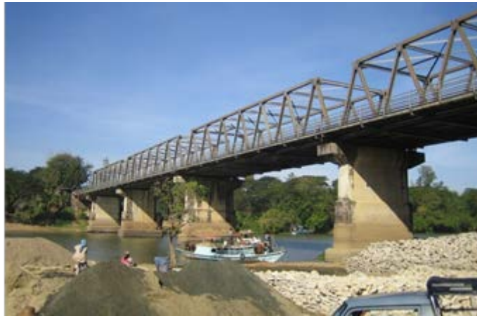
Photo—4.1 Kyaunkong Bridge
