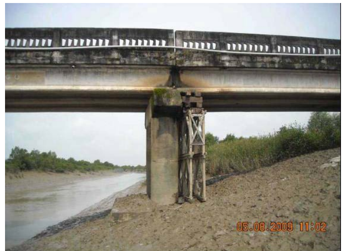
Photo-4.5 Temporal installed support
