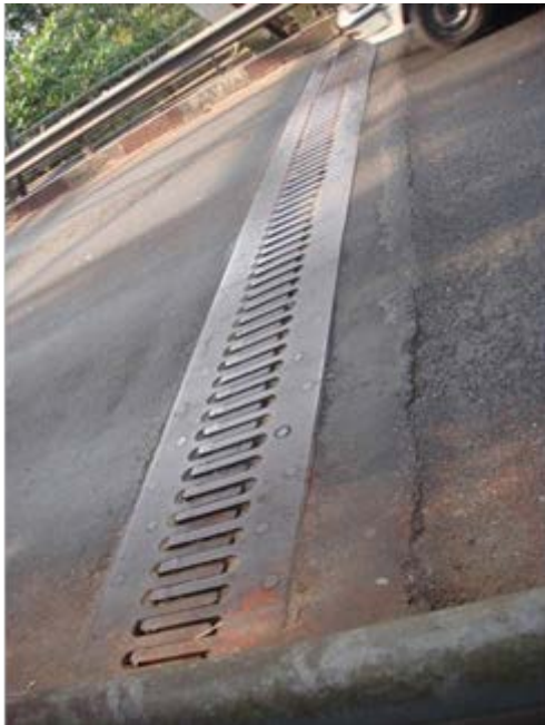
Photo-4.11 Expansion joint (Yangon side)
