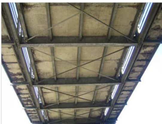
Photo—4.2 Concrete slab of Kyaunkong Bridge
