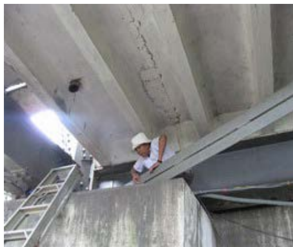
Photo-5.2 Slab of Bayinaung Bridge (Type II)
