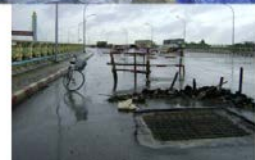
Photo-4.53 Slab under repairing
