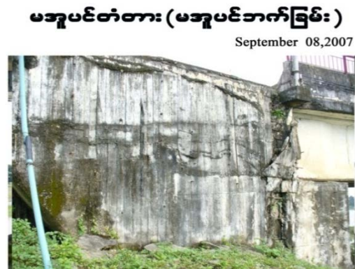
Photo-4.29 Abutment (Maubin side)
