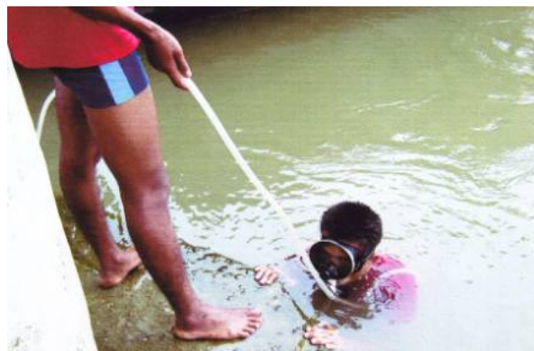
Photo-3.16 Survey of pile in the water
