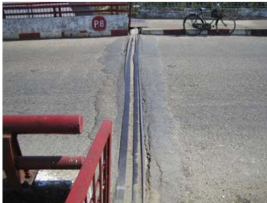
Photo-4.28 Expansion joint (Maubin side)
