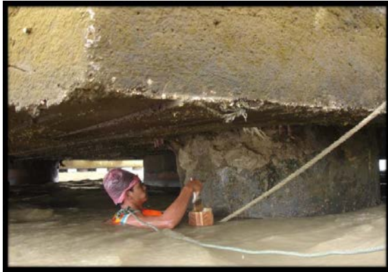
Photo-3.13 Repair of pile top
