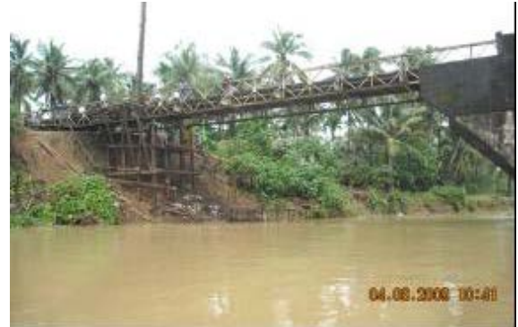
Photo-3.4 Subsequent flooding washed away the temporary bridge pier and traffic was halted
