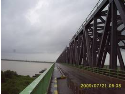
Photo-4.6 Thanlyin Bridge
