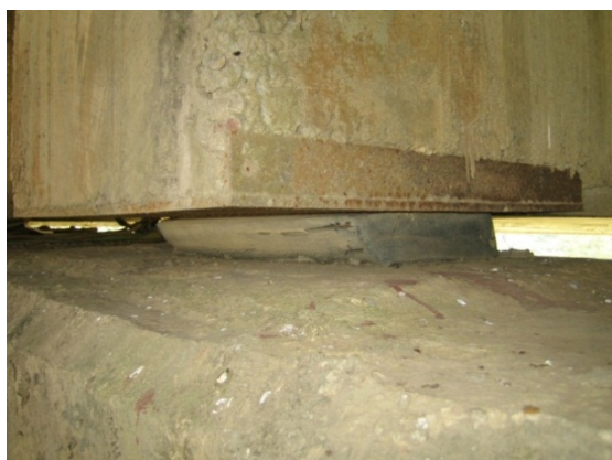
Photo—4.25 Rubber shoe subject to major shear deformation
