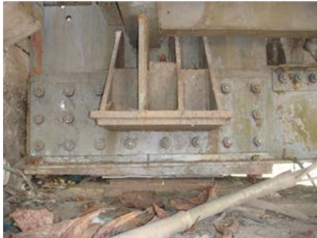
Photo—4.10 Movable shoe (Yangon opposite shore side)
