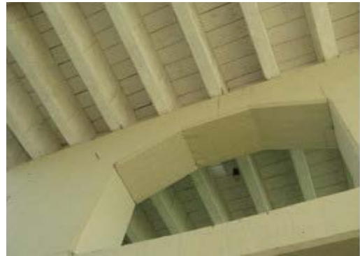
Photo-4.58 Slab of an approach concrete bridge
