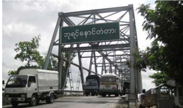
Photo-4.8 Bayinaung Bridge
