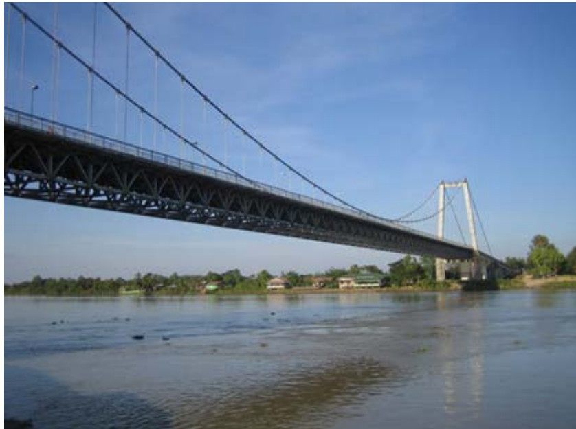
Photo—4.71 Pathein Bridge
