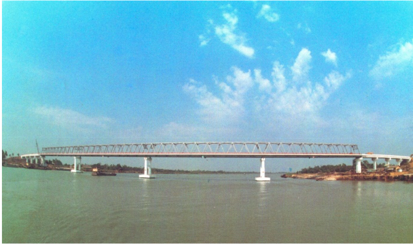
Photo—4.24 Maubin Bridge
