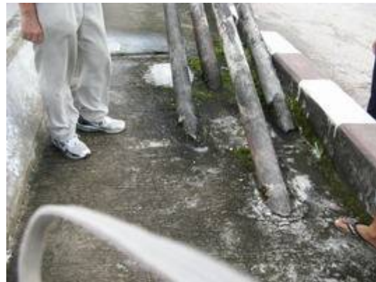
Photo-4.22 Cable passes through the road surface
