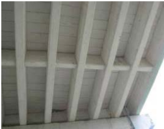
Photo-5.1 Slab of concrete girder bridge (Type I)
