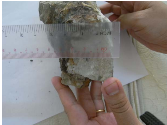
Photo—4.62 Rebar corrosion and concrete covering
