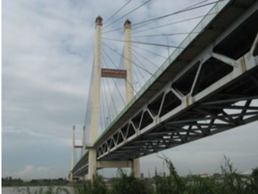
Photo-4.41 Aunzaya Bridge
