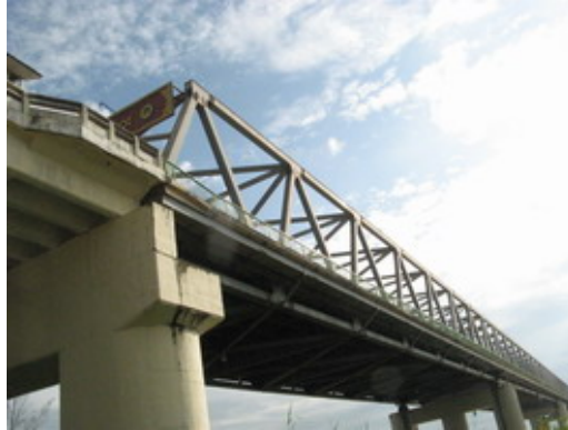
Photo—4.54 Shwe Pyithar Bridge
