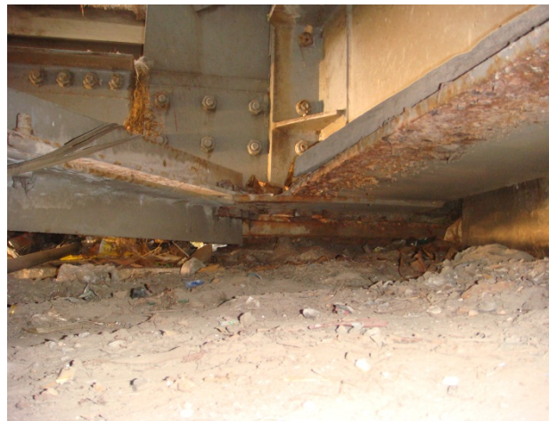
Photo—4.9 Movable shoe (Yangon side)
