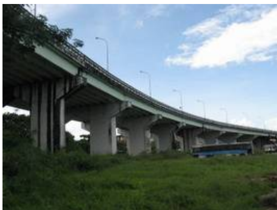
Photo-4.52 Approach concrete bridge of Mahar Bandoola Bridge
