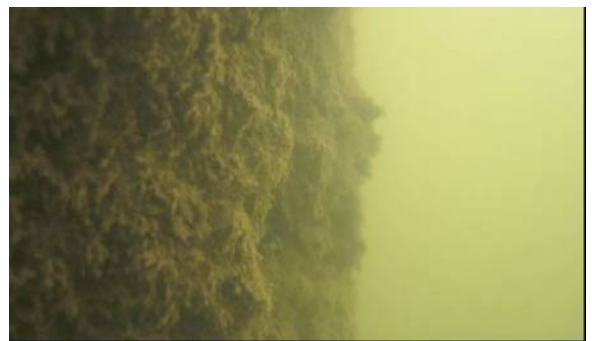
Photo-3.17 Pile in the water
