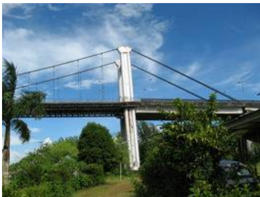
Photo-4.19 Inclined tower
