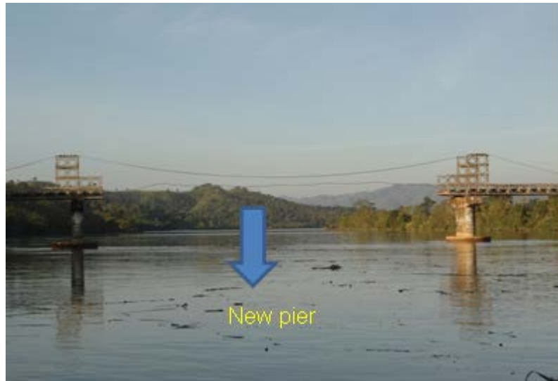
Photo—4.40 Da let-Chaung Bridge under repairing
