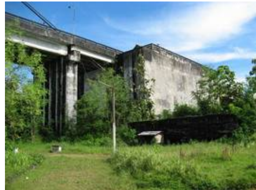
Photo-4.18 Anchorage (south side)
