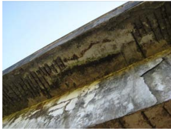
Photo—4.66 Underside of an approach concrete bridge's walkway
