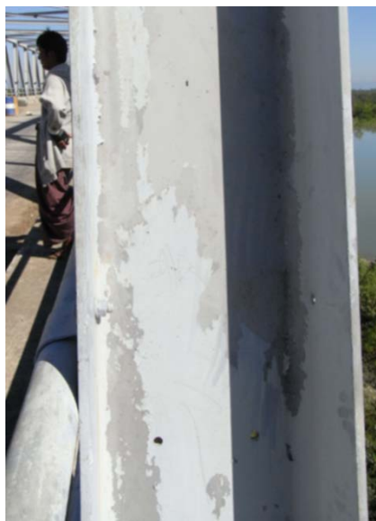
Photo-4.69 Peeled paintwork of the truss
