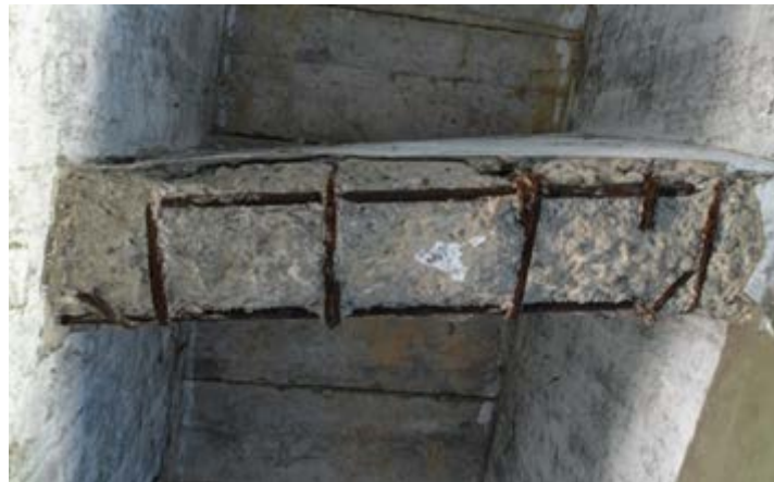
Photo—4.67 Cross beam of an approach concrete bridge
