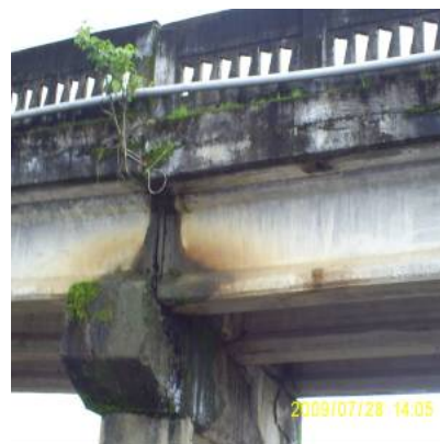
Photo-3.2 Concrete girder nearly from substructure
