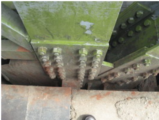
Photo-4.15 Panel point of truss
