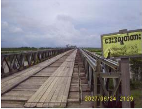
Photo-3.7 Bailey girder bridge
