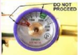
Checking gas pressure
