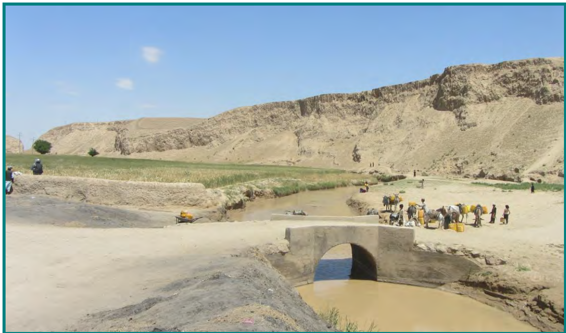
Figure 1.2. Irrigation channel, fed by water drawn from the River Shirin Tagab, near Araba, Dowlatabad District. Photo taken by DACAAR on 12 th May 2013.
