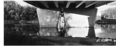
Victoria Street overpass, 2010
