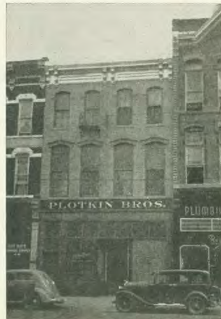
The Building on Larimer Street in which was established by Dr. Auguste Renouard the first school of embalming in the United States
