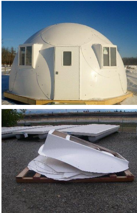
Diagram 3. View of disassembled and assembled InterShelter™ Domes and interior plan
