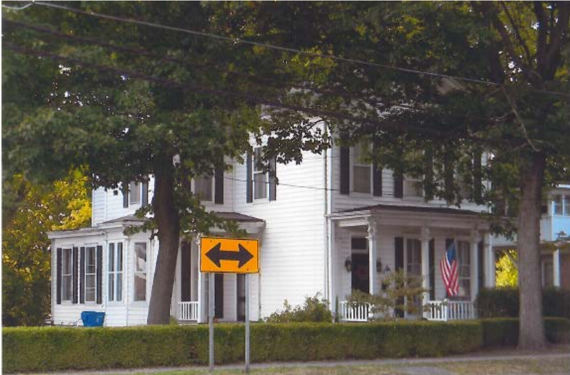
Figure 14: Survey Update Photo of 205 S. First, Fairfield, IL, 2017
