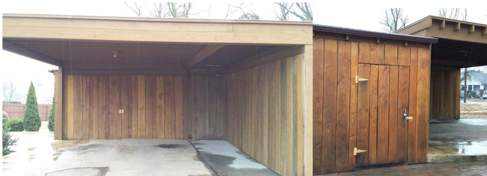
Non-contributing carport. Photograph on the left is facing east (yellow arrow); photograph on the right is facing southwest (red arrow).
