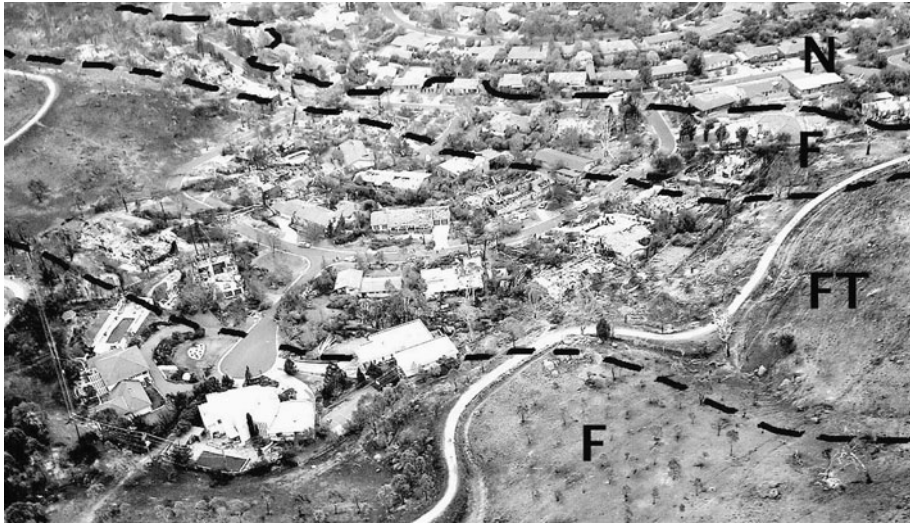
Fig. 7 Aerial post-fire photograph of Lincoln Close, Chapman. A mix of damage types is evident— F fire only, FT fire and tornado, N none. This view to the north-west is from just north of Mt Arawang
