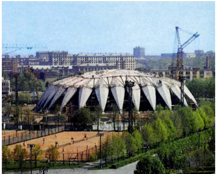
Druzhba Multipurpose Arena under construction
